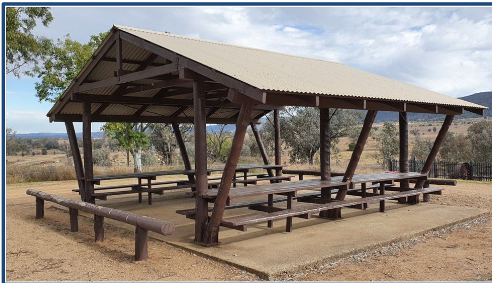
Figure 14 - Assets Sheltered picnic area with seating, benches and concrete slab floor.
