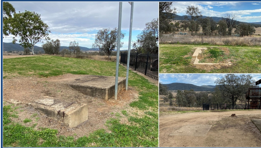
Figure 17 - Assets Various concrete mine shaft cappings or pads for infrastructure demonstrate the history of mining at All Nations Hill.
