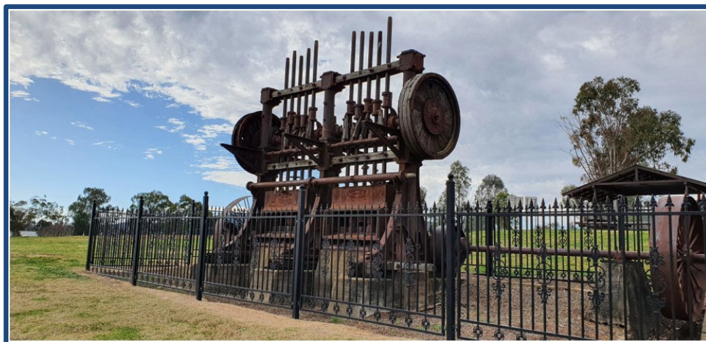
Figure 13 - Assets Metal enclosure fencing erected on the perimeter of the Stamper Battery site.
