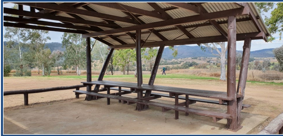
Figure 15 - Assets Inside the sheltered picnic area.
