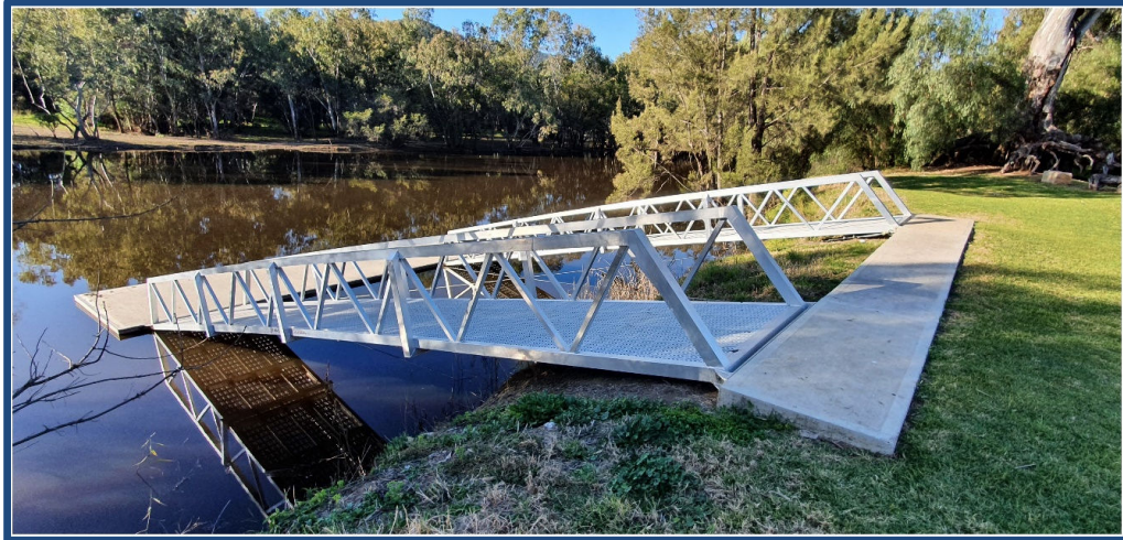
Figure 21 – Assets - Instream Structure: Floating Pontoon, located at Riverside Picnic Area
