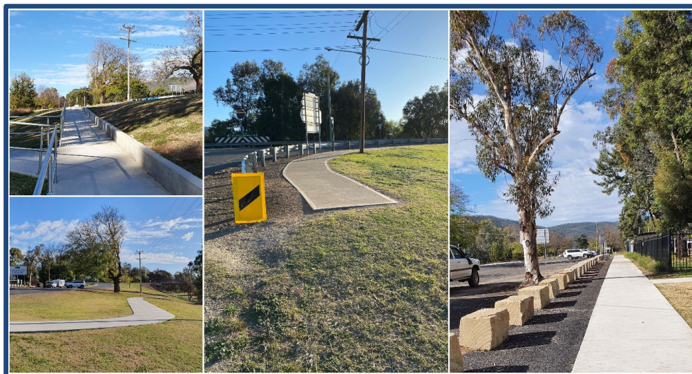
Figure 23 – Assets - Concrete Pedestrian Pathways Access to Riverside Picnic Area from Copeton Dam Road and Campbell Bridge (left and centre); Pathway to car parking area and neighbouring Caravan Park.
