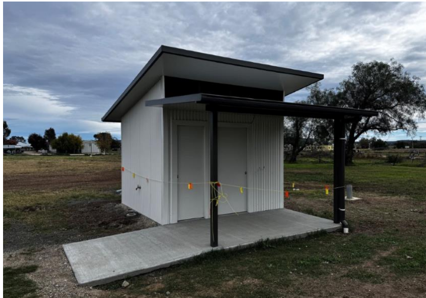
Warialda Rail Recreation Ground Amenities
