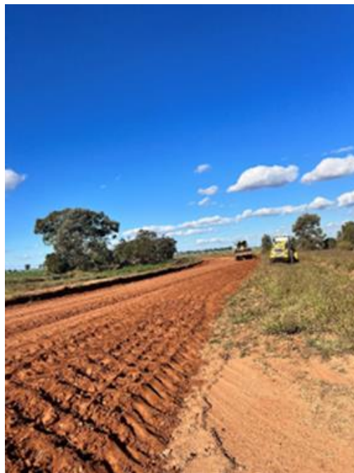
SR9 IB Bore Road
