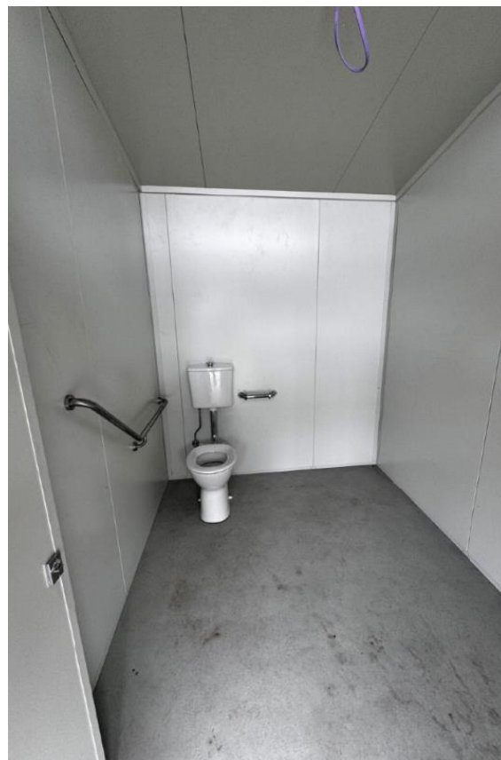
Warialda Rail Recreation Ground accessible toilet
