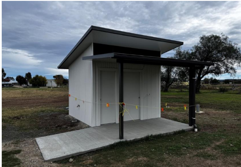
Warialda Rail Recreation Ground Amenities
