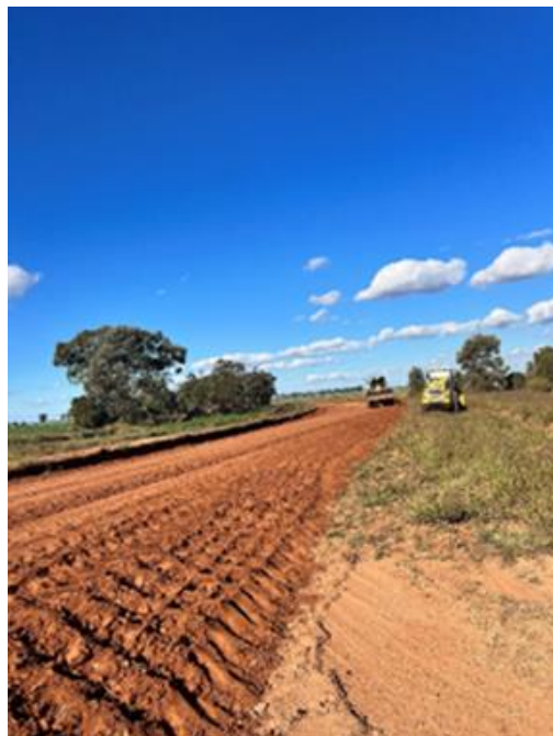
SR9 IB Bore Road
