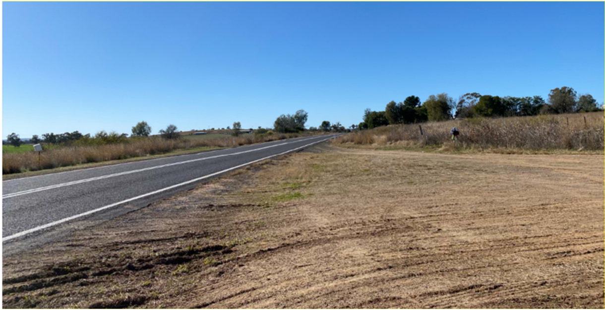
Figure 11: View from Glen Royal property entrance looking east along Gwydir Highway
