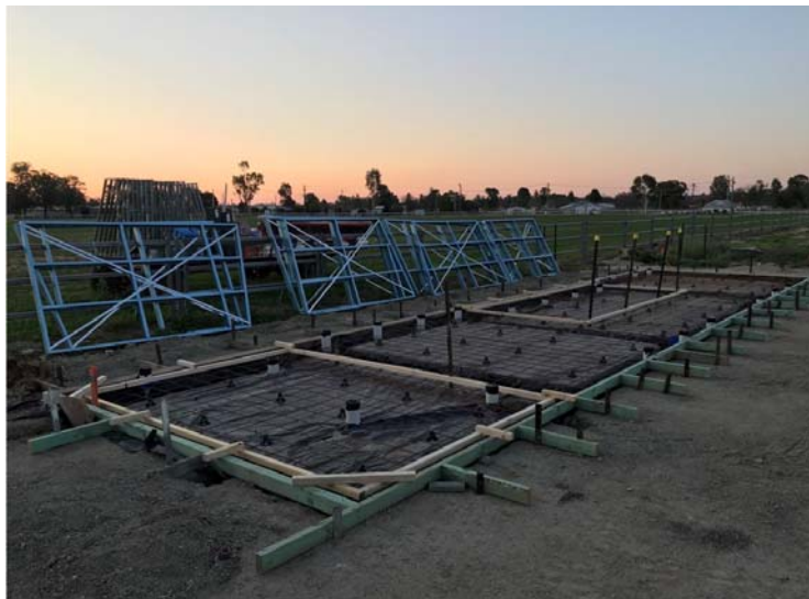
Bingara Showground Amenities – footings and slab framework
