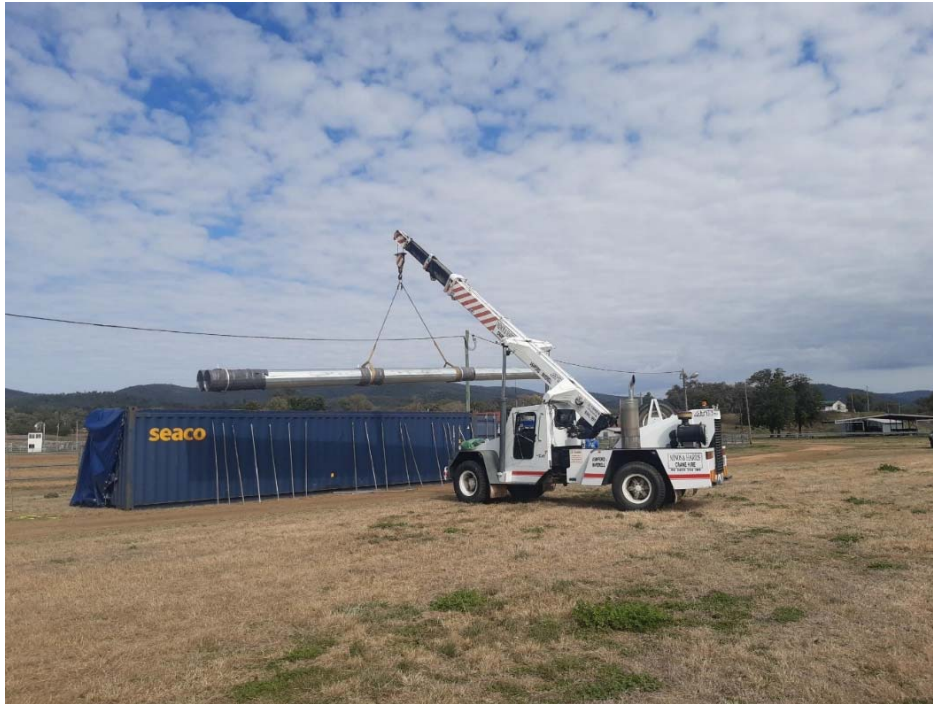
Unloading the light pole towers, Bingara Showground
