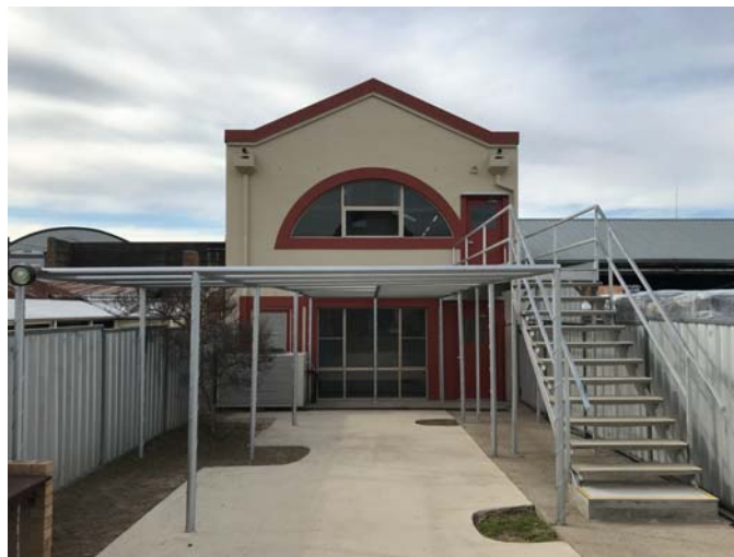
Rear view at 47 Hope Street Warialda
