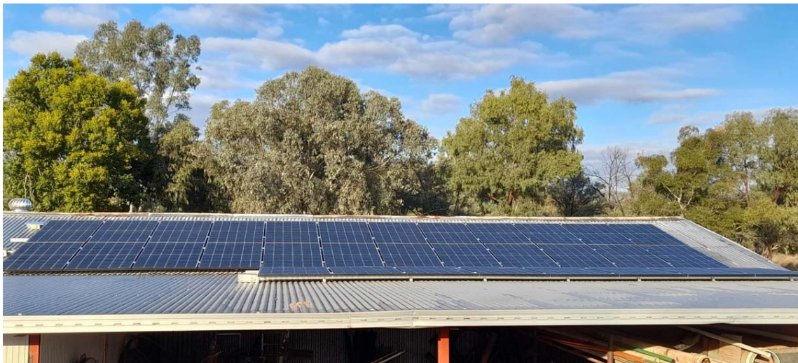
New solar panels on the roof of the Sewerage Treatment Plant, Bingara
