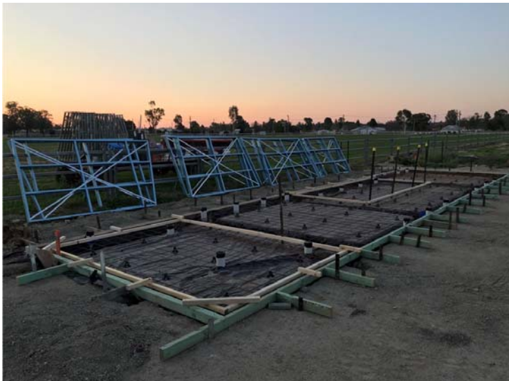
Bingara Showground Amenities – footings and slab framework
