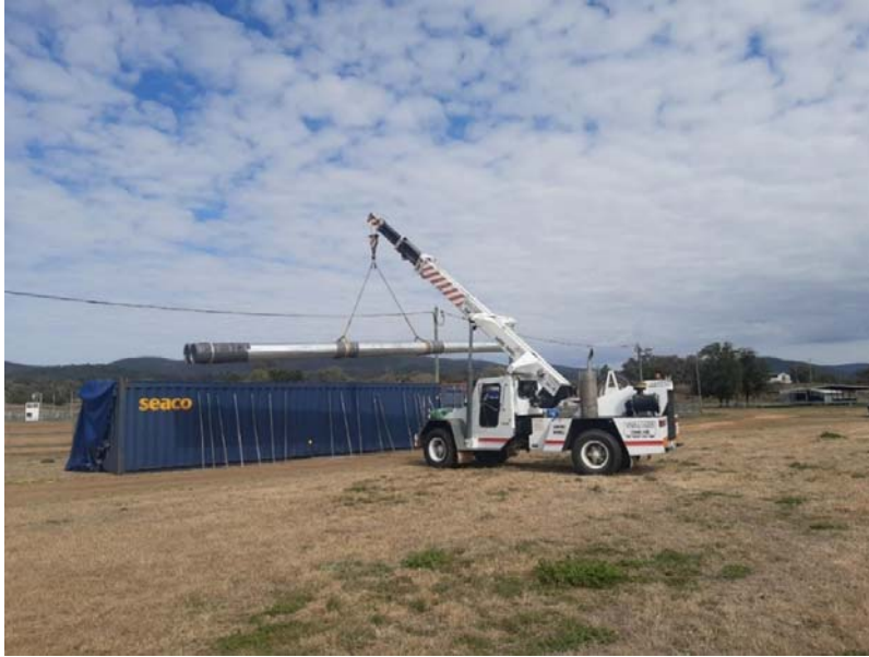
Unloading the light pole towers, Bingara Showground
