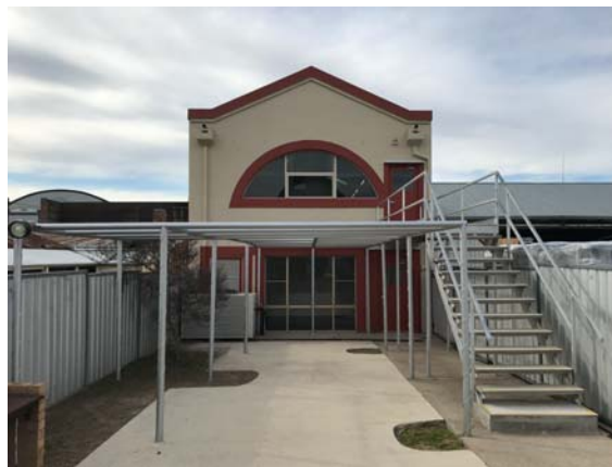
Rear view at 47 Hope Street Warialda
