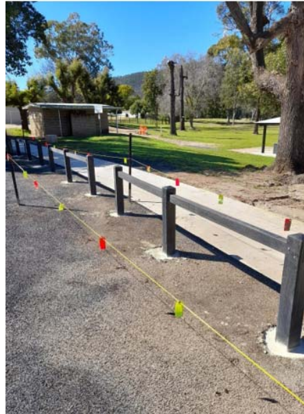
New barrier at car park, Cunningham Park
