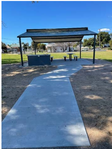
A new path to new shelter, BBQ and tables at Captain Cook Park
