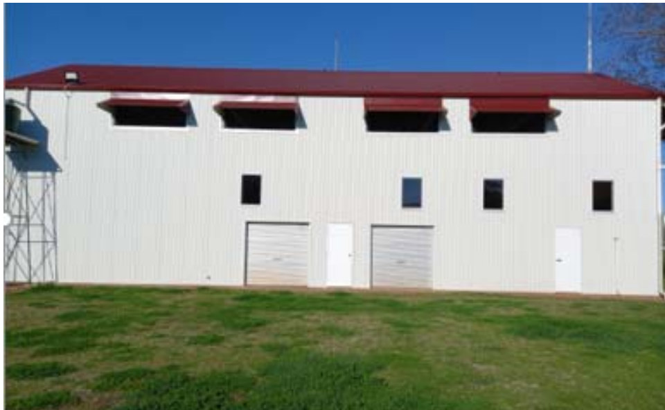
Work on Showground Grandstand is expected to be completed in September
