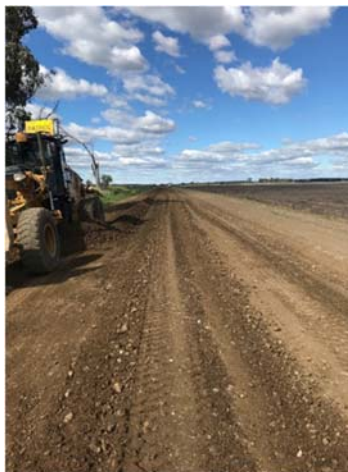
Material with Polycom being re-laid for SR13 Oregon Road pavement upgrade.
