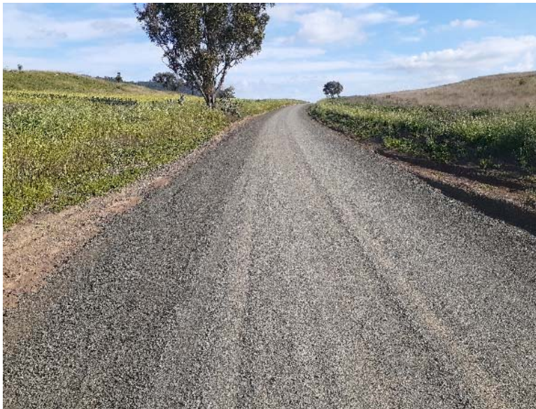
SR45 Bereen Rd Resheeting
