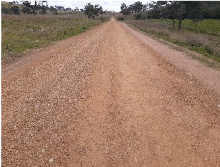
SR54 Pinecliff Rd Resheeting
