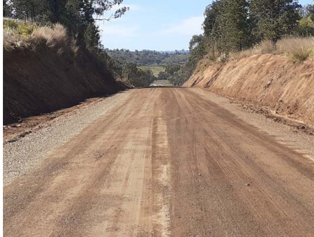
Horton Road Earthworks
