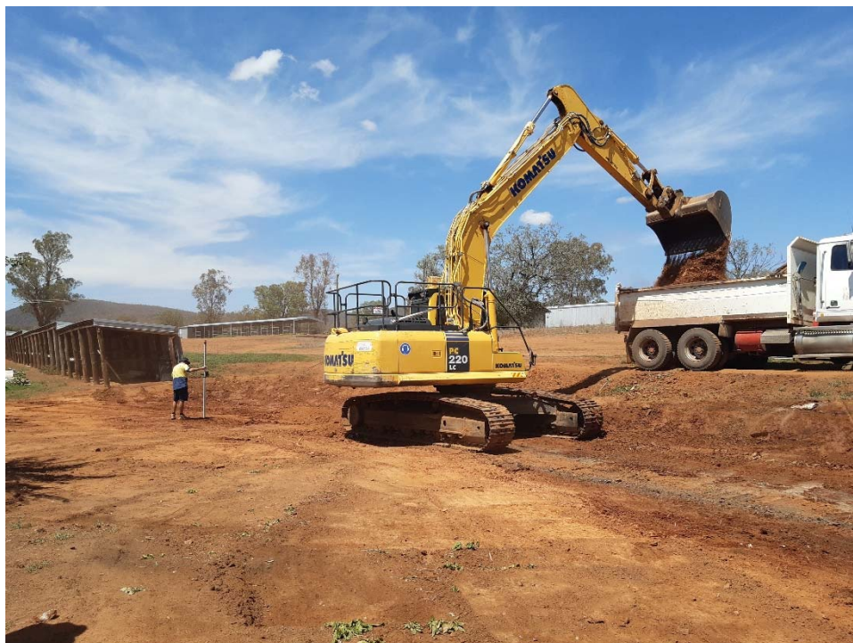
Excavation of site for new multi-purpose pavilion
