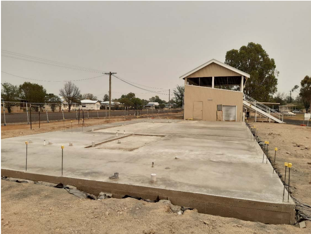
New amenities slab at Gwydir Oval, Bingara
