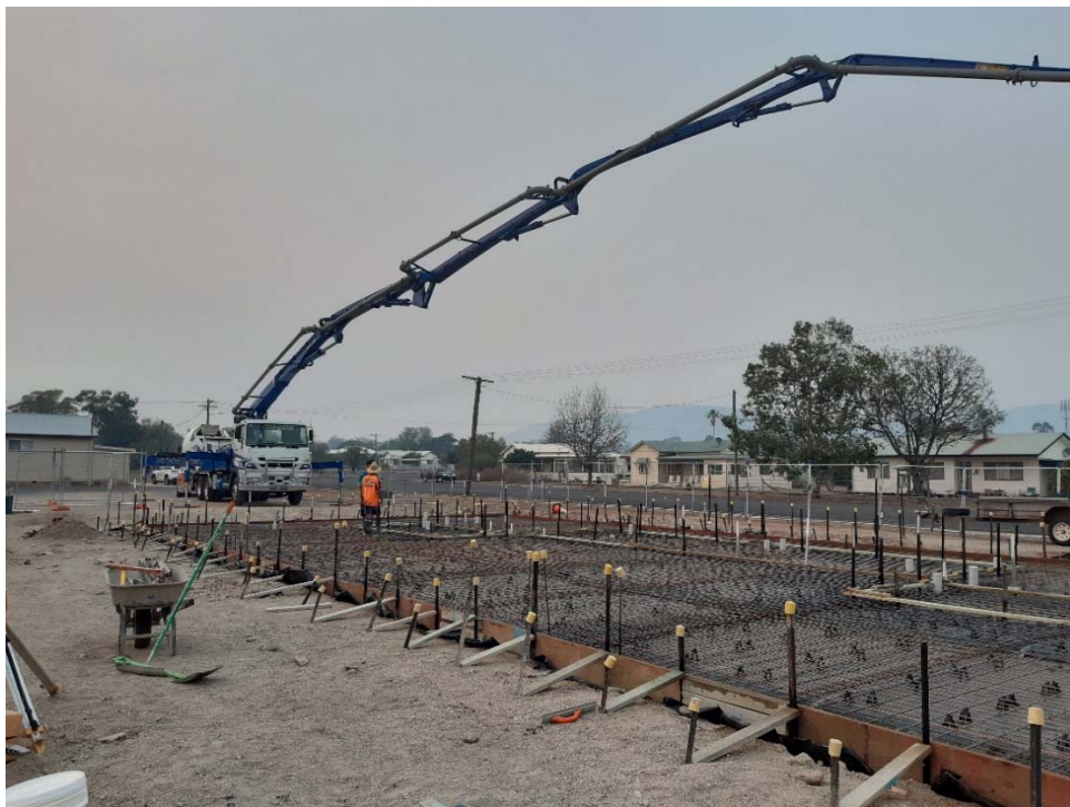
Formwork for the new amenities slab at Gwydir Oval, Bingara
