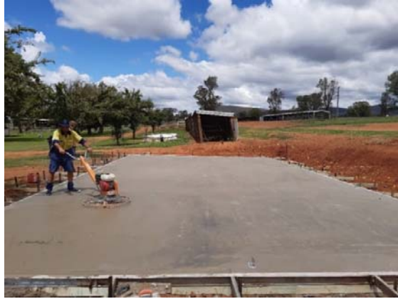
Slab for the Bingara Showground multi-purpose pavilion
