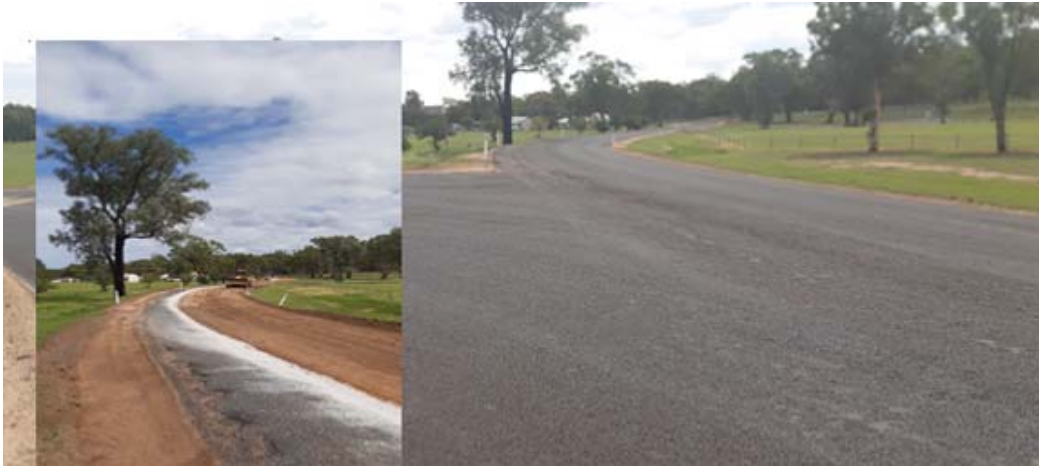
Mosquito Creek Road / Long Street stabilisation
