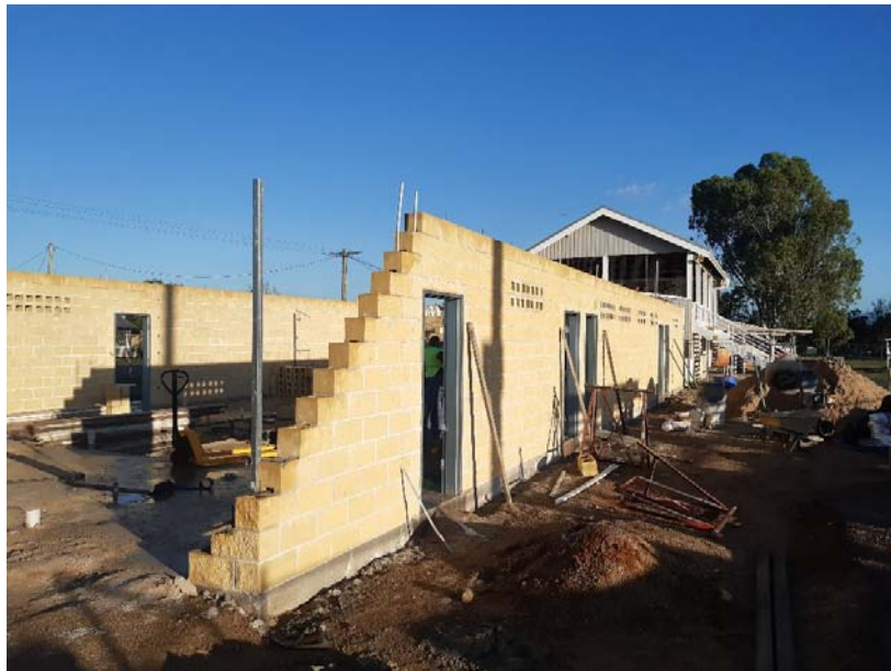
Work on the Gwydir Oval Amenities block
