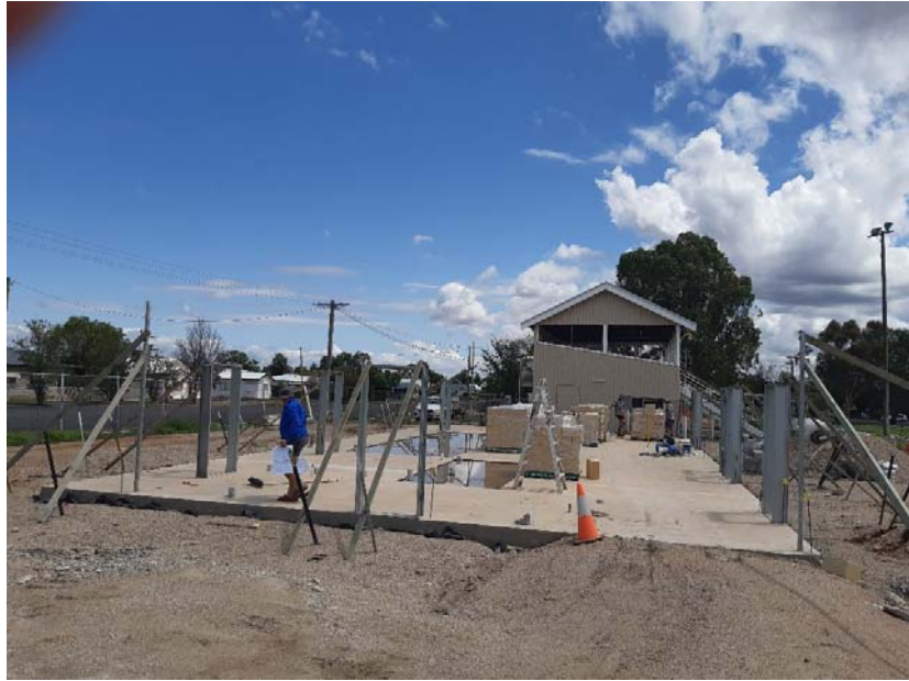
Gwydir Oval – start of block laying
