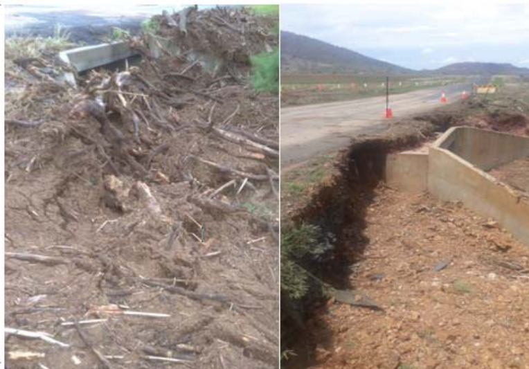
MR133 Killarney Gap Road Dry Creek Causeway
