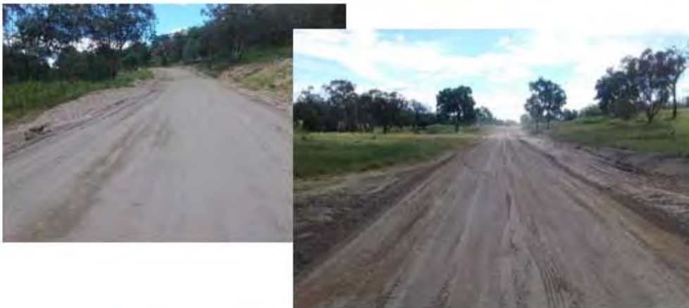
Wearnas Road - 5km Section completed in the Beehive Mountain area
