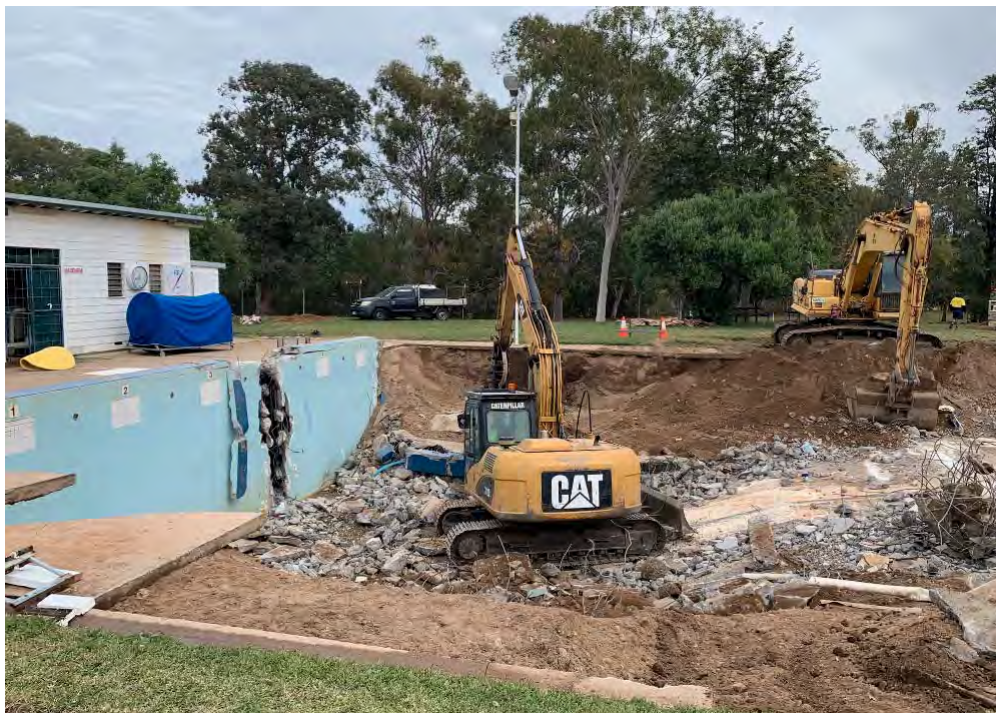
Removing the Bingara pool
