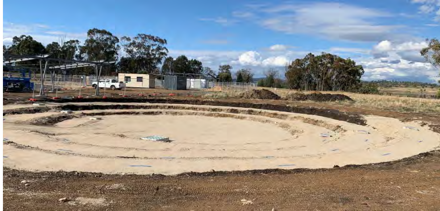
The Amphitheatre at the Myall Creek Memorial site
