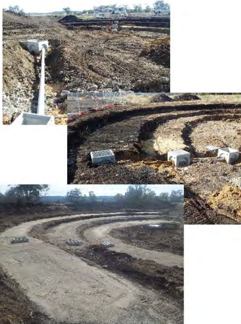
Works in progress at the Myall Creek Memorial Site
