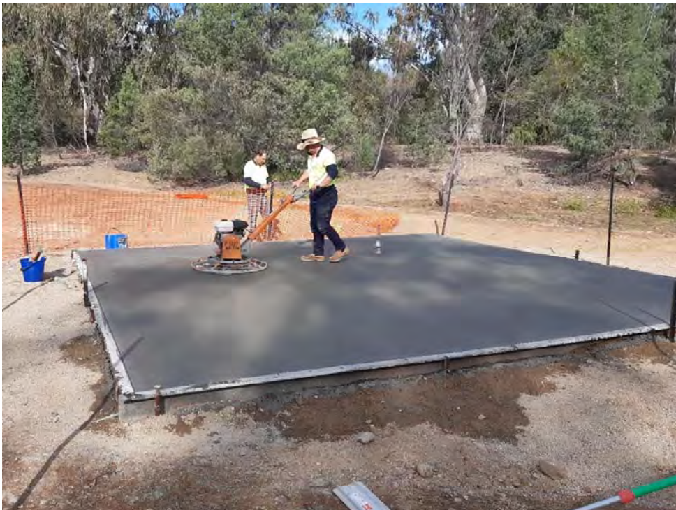
Bingara Anglers Club shelter slab – near boat ramp
