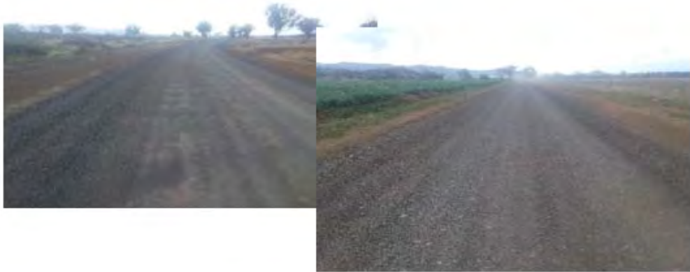
Caroda Road - 6.32km section is completed between "Killara" and "Reata"
