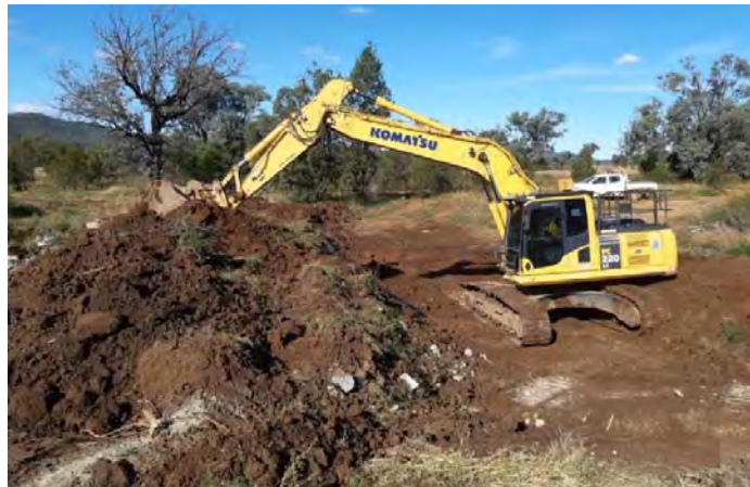
Working on the 'leaky dam' project at TLC
