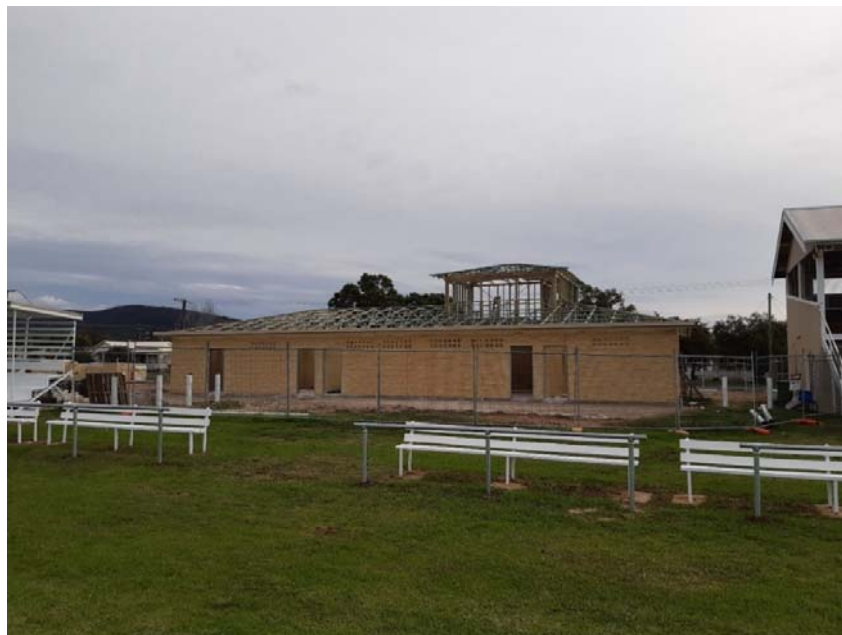
Gwydir oval new amenities building
