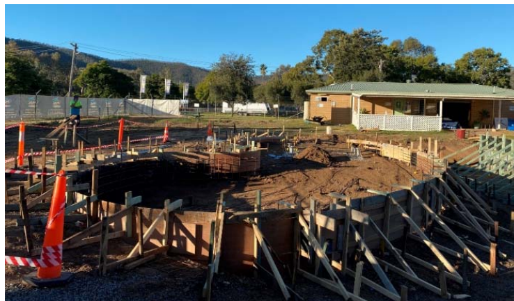
Splash Program Pool formwork
