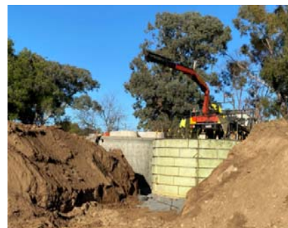
Installation of screw piers (left) and onsite construction of underground pool tanks (right)
