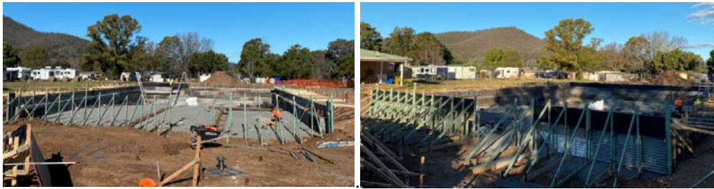
Pool formwork (before and after)
