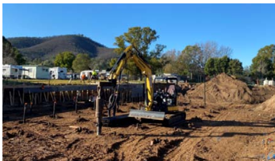
Installation of screw piers (left) and onsite construction of underground pool tanks (right)
