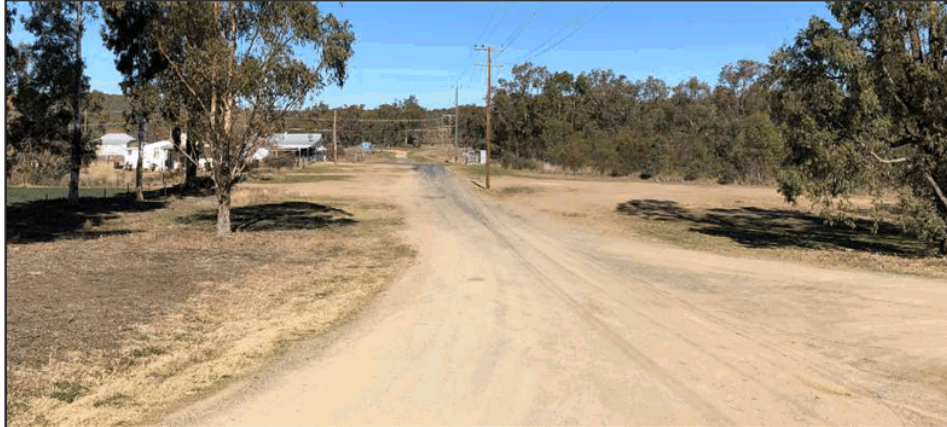
Figure 5: West Street looking south along power line corridor with cleared link to Gwydir Highway
