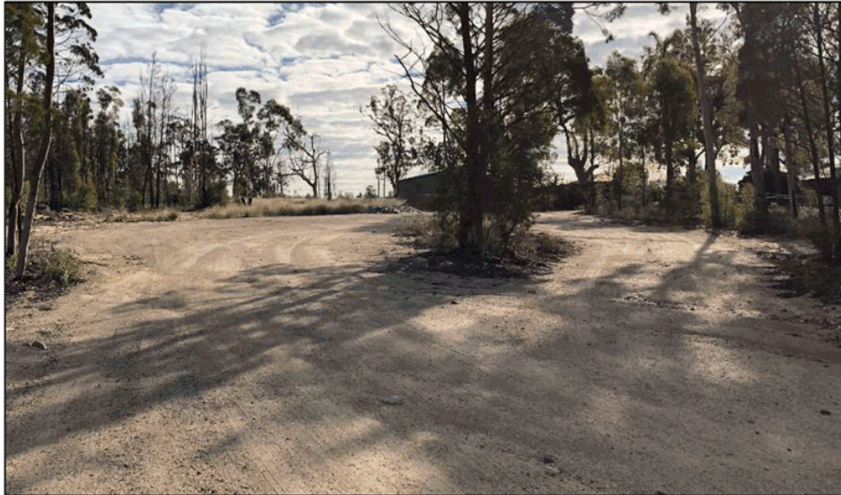
Figure 11: Clear zone to south of southern residence in Plunkett Street.
