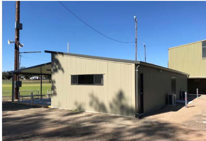
Rear view of the Function Centre
