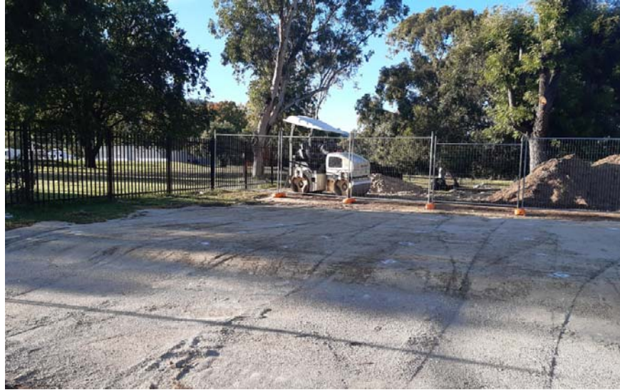
Cunningham Park new toilet block pad
