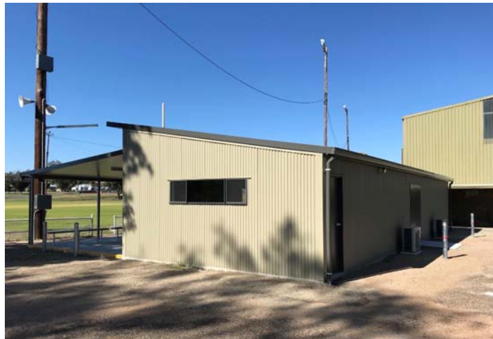
Rear view of the Function Centre
