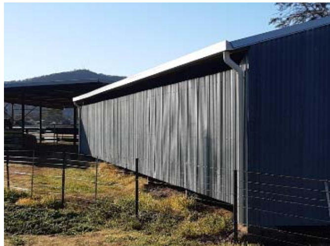
Bingara showground bull shed – gutter replacement
