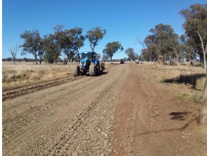
SR31 Eulourie Road, Gravel Resheeting
