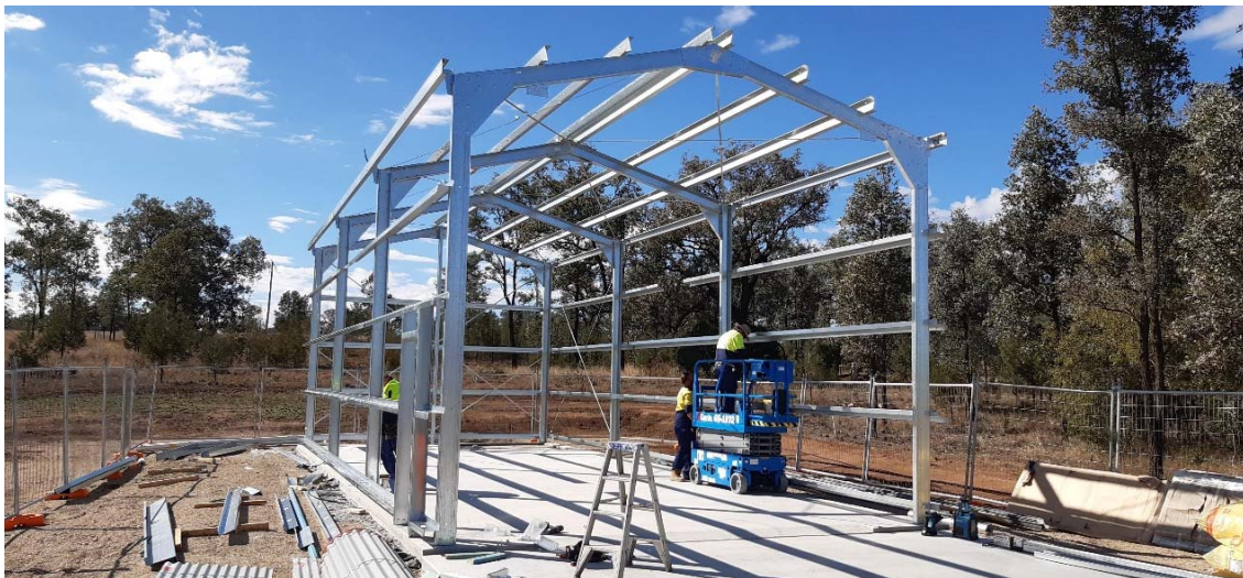
Gineroi RFS Shed Construction
