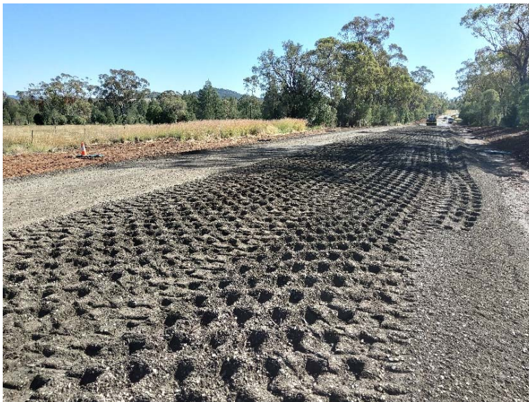
Work on the Linwood segment of MR63
