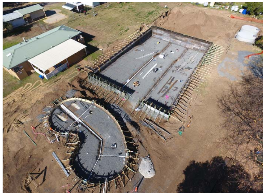
Drone view of the Bingara Pool progress
