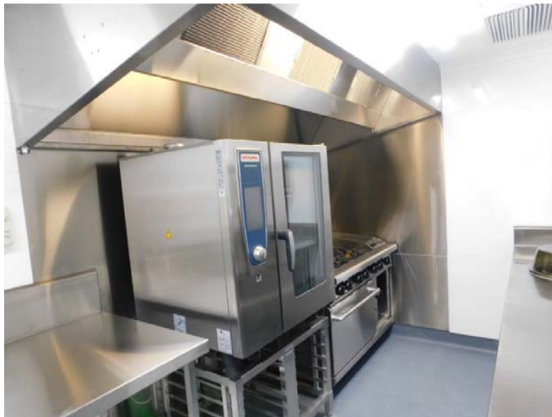
Images of the renovated kitchen at Naroo
