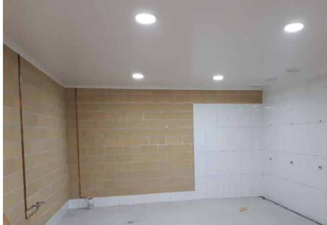
Tiling in the Gwydir Oval Amenities building
