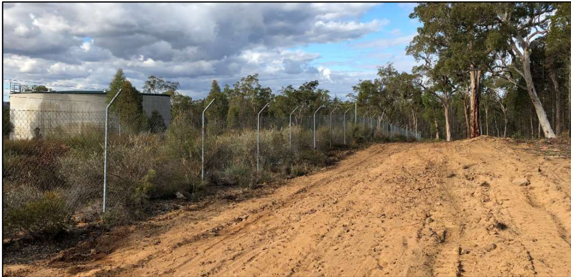
Figure 10: Southern fence of Southern Reservoir showing shrub growth within the reservoir compound.
