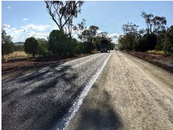
MR63 Linwood Construction
