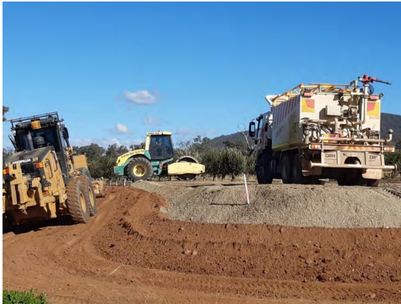
Building the pad for the Interpretive Centre at TLC
