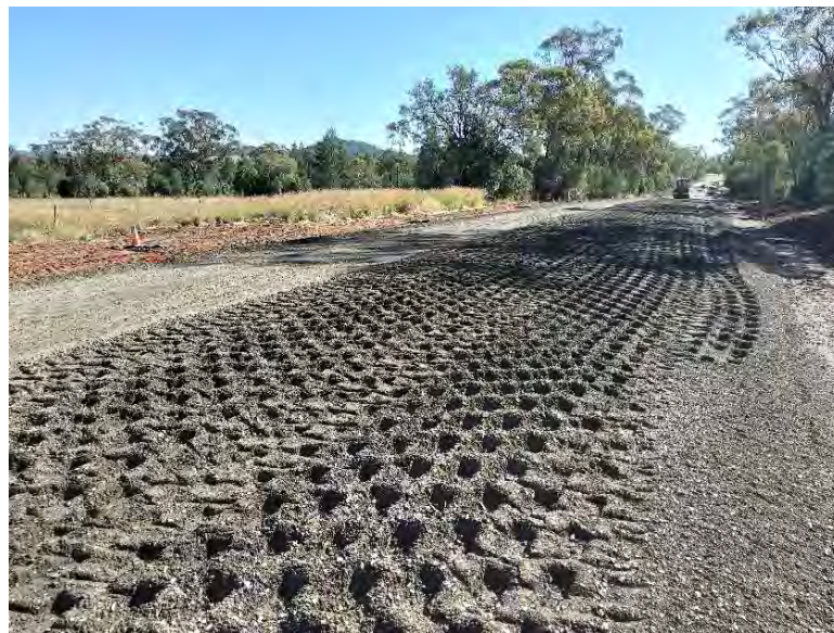
Work on the Linwood segment of MR63
