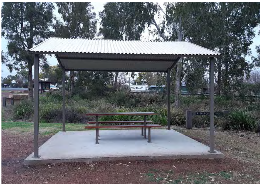
Junction Park, Bingara Shelter
