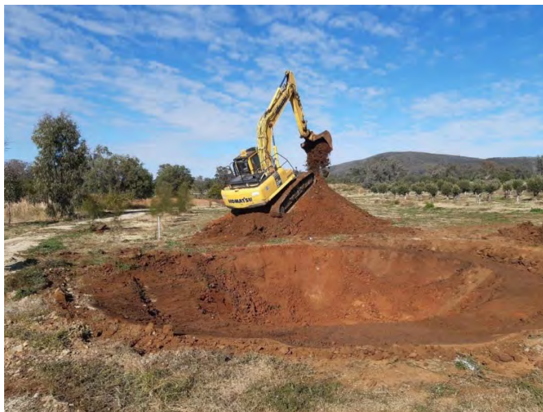
Working on the spiral hill and hollow project at TLC
