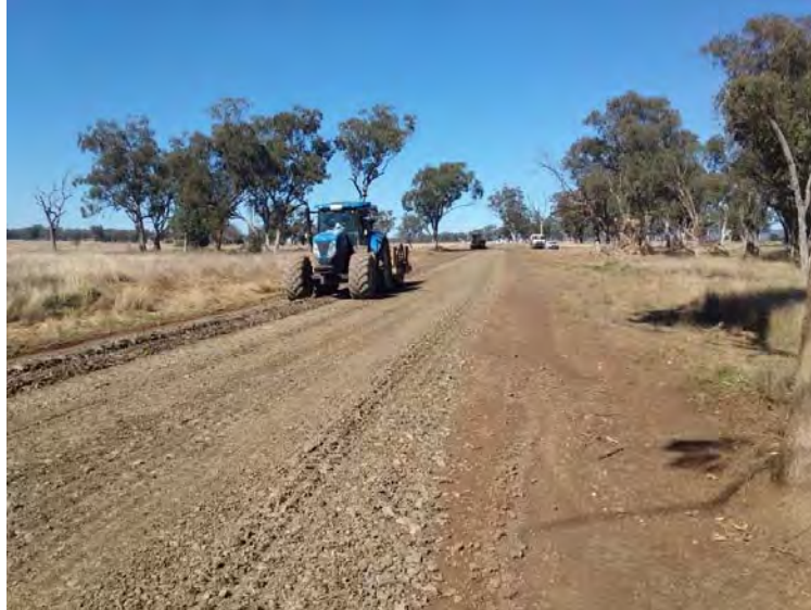
SR31 Eulourie Road, Gravel Resheeting
