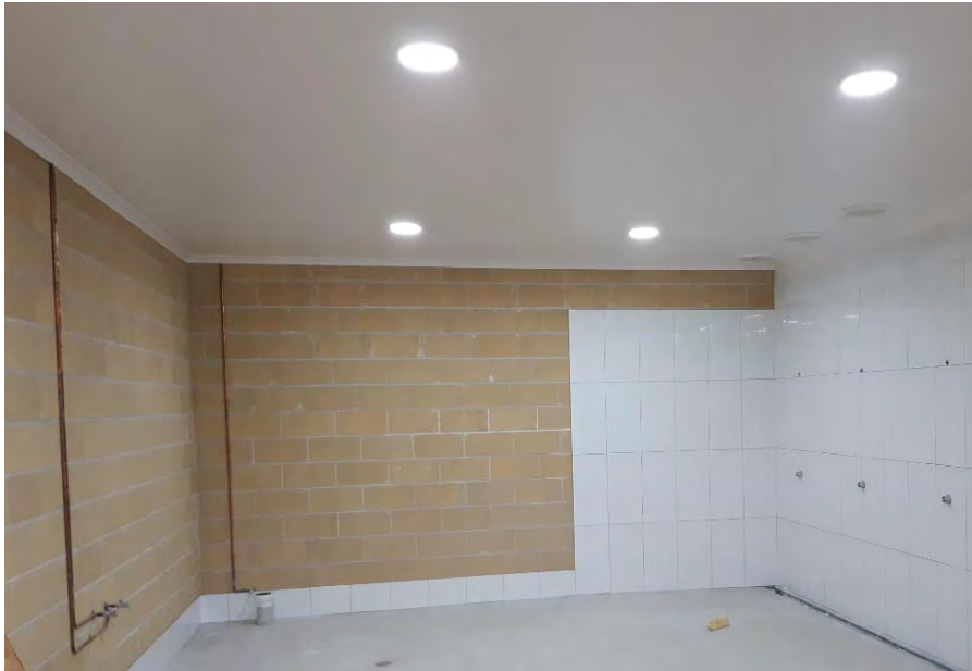
Tiling in the Gwydir Oval Amenities building
