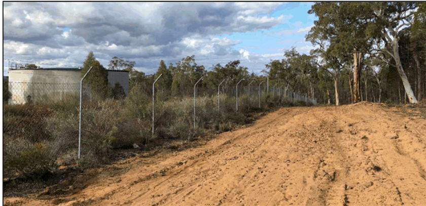
Figure 10: Southern fence of Southern Reservoir showing shrub growth within the reservoir compound.
