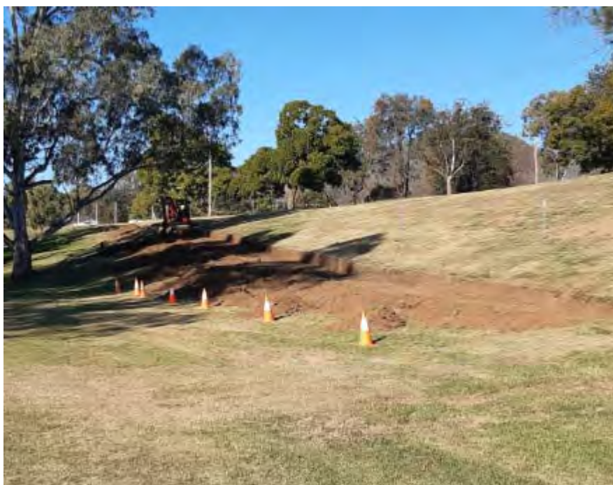
Footpath earthworks leading to the pontoon on Gwydir River
