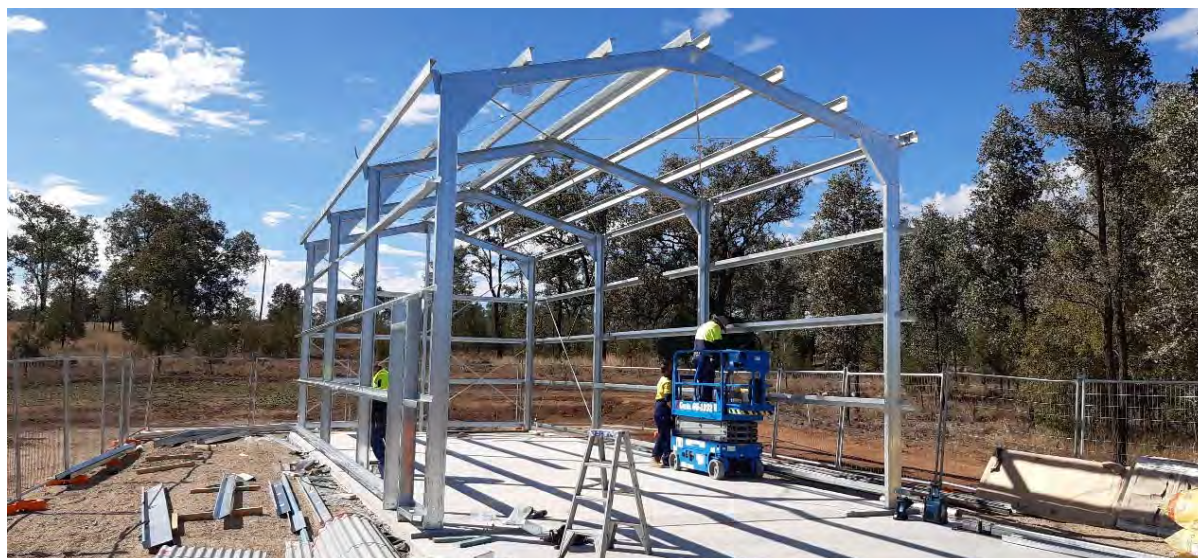
Gineroi RFS Shed Construction
