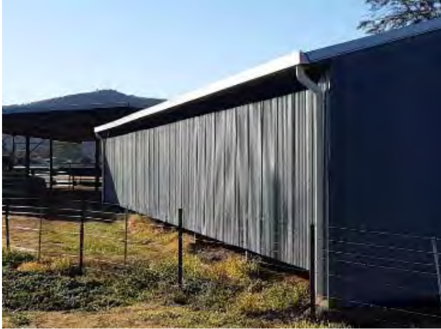
Bingara showground bull shed – gutter replacement
