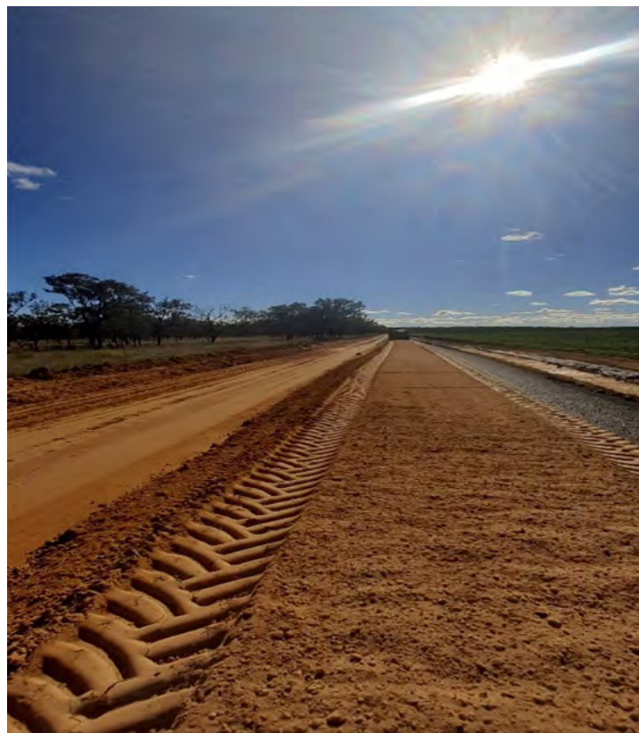
North Star Road – Flaggy, Stabilising
