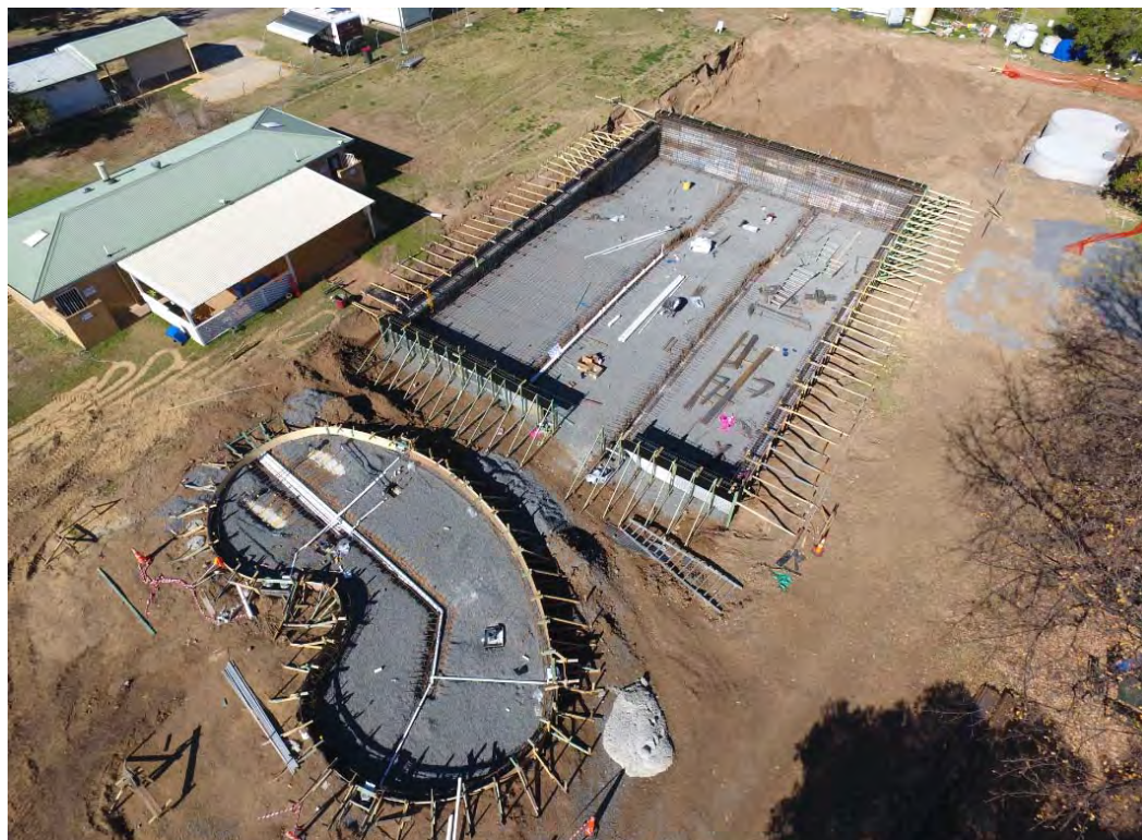
Drone view of the Bingara Pool progress
