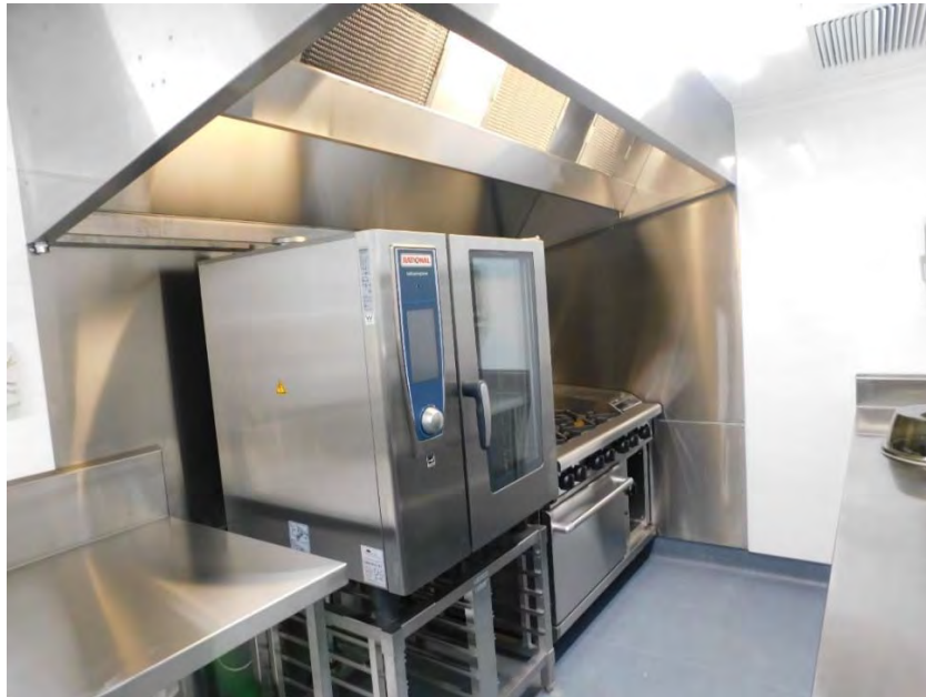
Images of the renovated kitchen at Naroo
