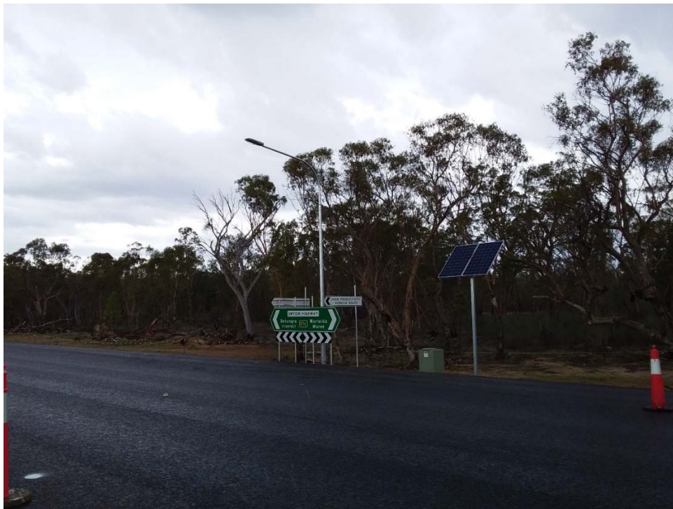
Gwydir Highway intersection signage and solar Light installation
