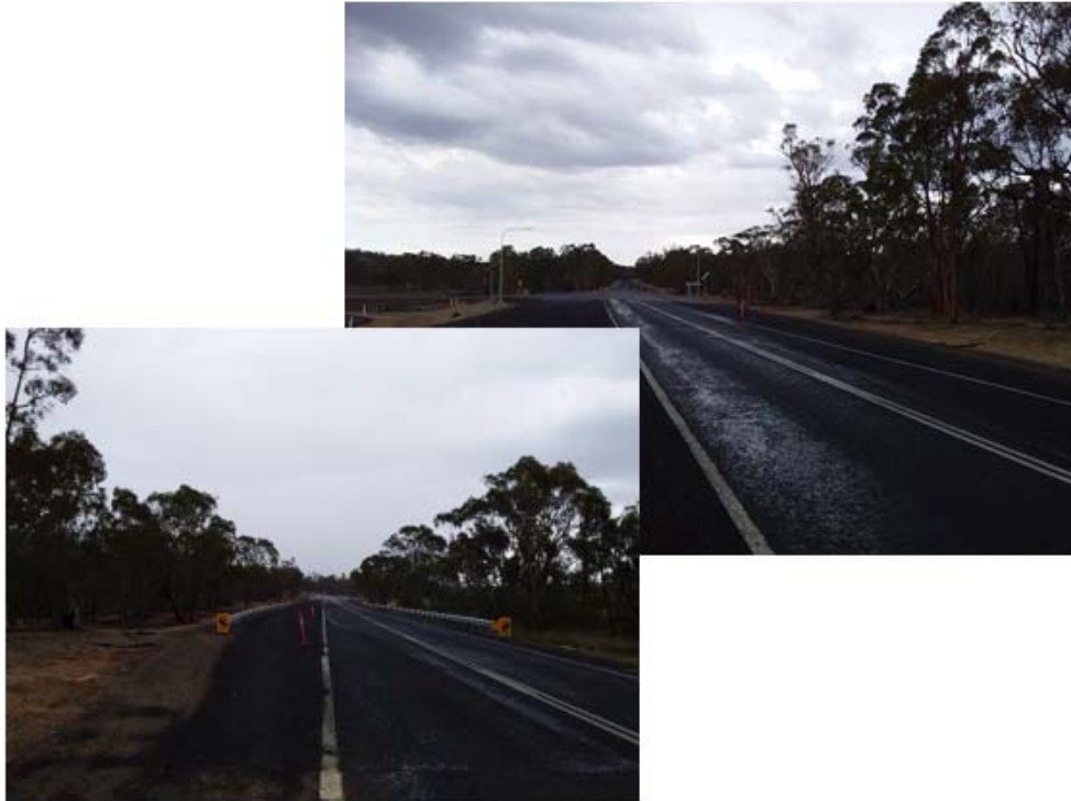
Gwydir Highway intersection works onto the Warialda HPV Route
