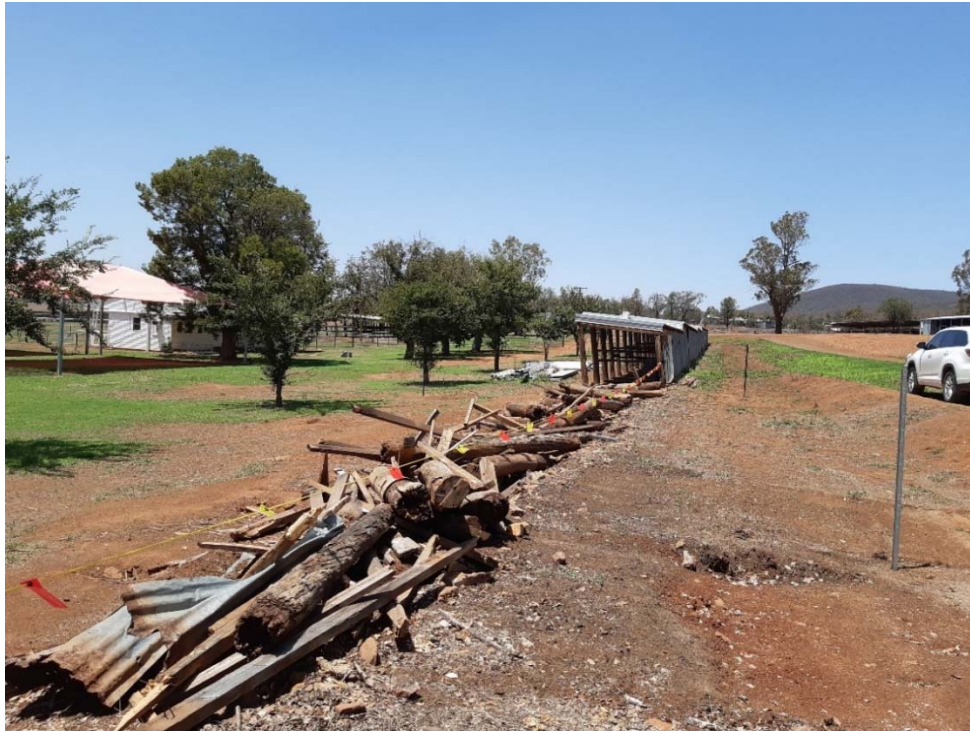
Removal of old stables at the Bingara Showground
