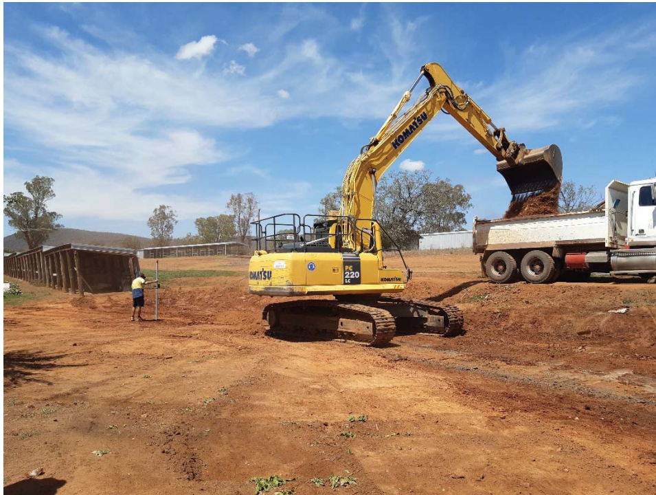
Excavation of site for new multi-purpose pavilion
