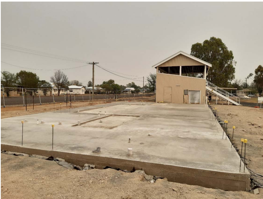
New amenities slab at Gwydir Oval, Bingara
