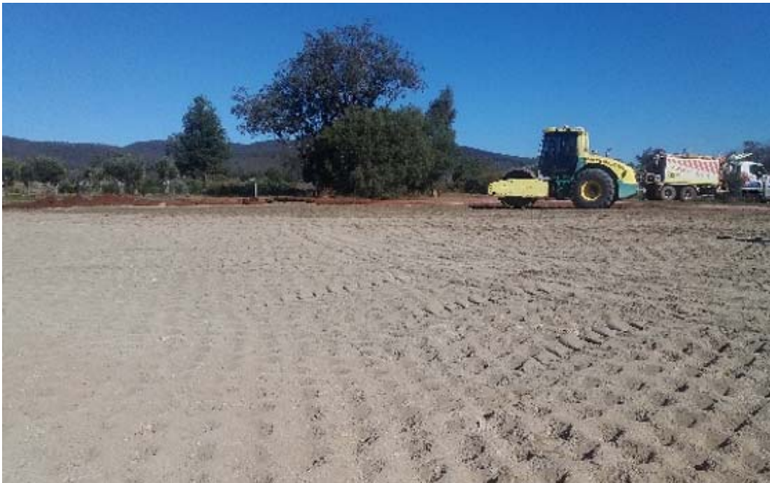
Earthworks at The Living Classroom
