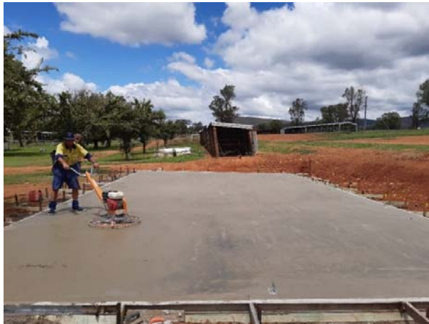
Slab for the Bingara Showground multi-purpose pavilion
