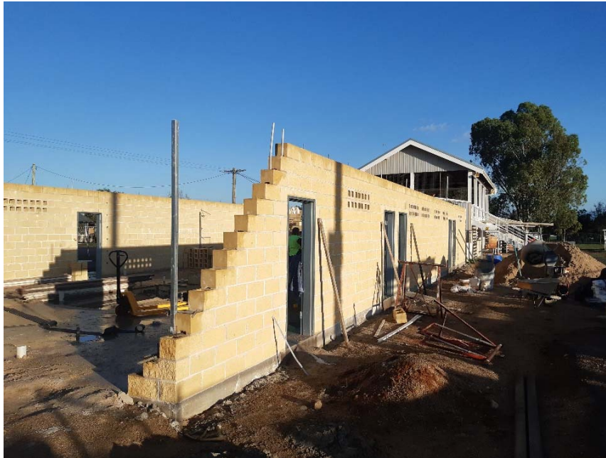
Work on the Gwydir Oval Amenities block
