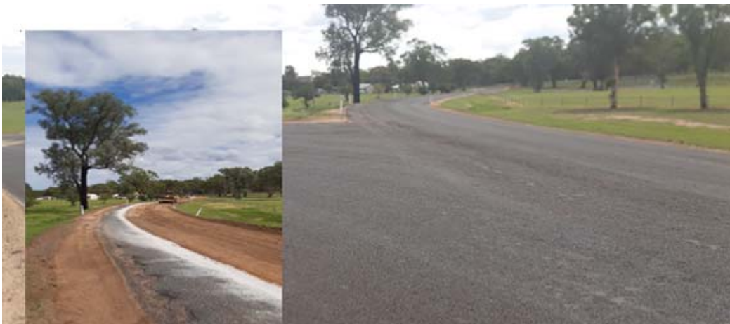
Mosquito Creek Road / Long Street stabilisation
