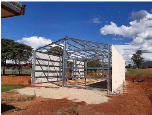
General Purpose shed at Bingara showground
