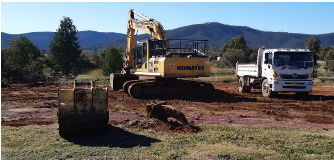
Preparation of the pad for the Interpretive Centre
