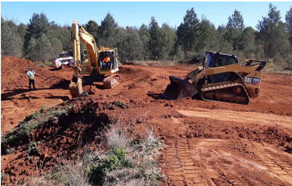
The training group remodelling the top dam at TLC
