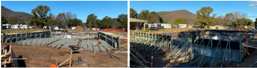
Pool formwork (before and after)
