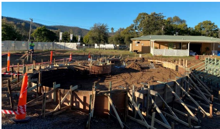
Splash Program Pool formwork
