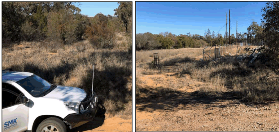
Figure 9: Photos of reserve areas around Warialda Substation on Warialda Road
