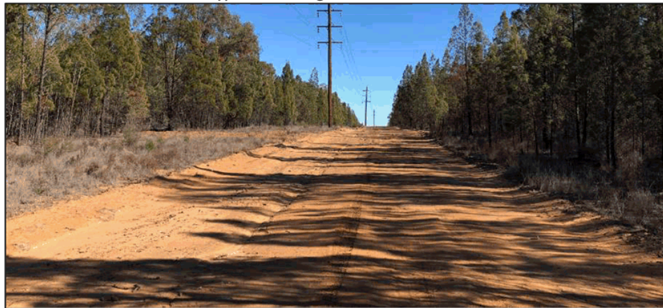
Figure 4: Typical clear zone along power line corridor. Historical fires have jumped this fire break due to low shrubs and cypress sucker growth within the corridor.
