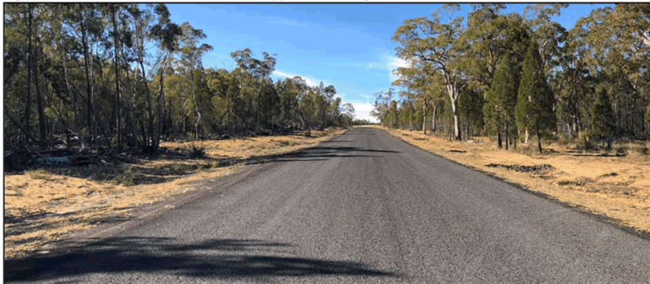
Figure 3: View of northern section of Bypass showing tall forest and clear zone
