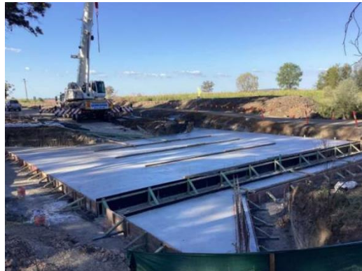
SR41 County Boundary Road, Gil Gil Creek
