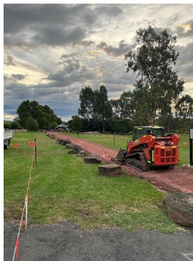
Footpath base preparation in Junction Park, Bingara.
