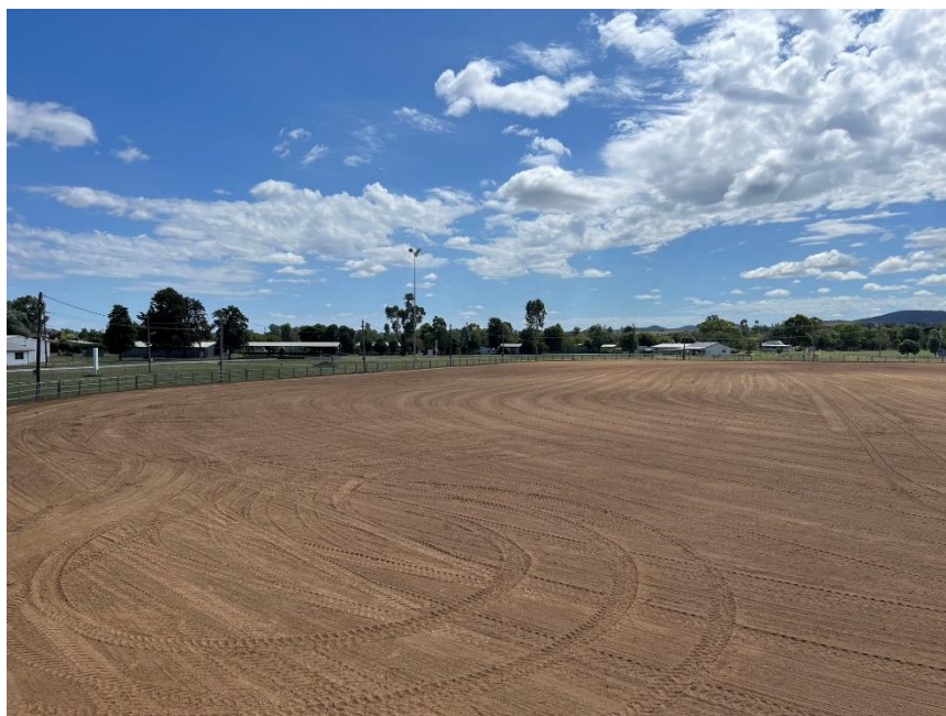
Bingara Showground laser levelling
