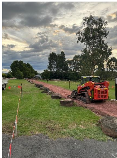
Footpath base preparation in Junction Park, Bingara.
