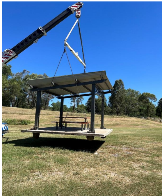
Moving the shelter down stream of Bingara Bridge
