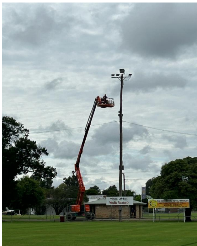
Repairs to Lighting at Warialda Recreation Oval
