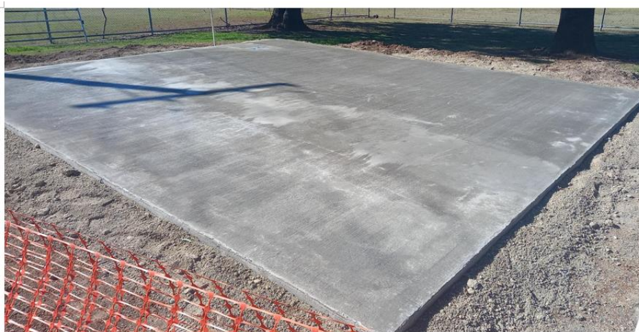
Slab for Swabbing Stall at Bingara Showground
