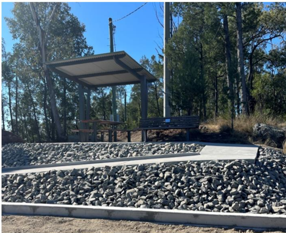
Batterham's Lookout picnic shelter and footpath
