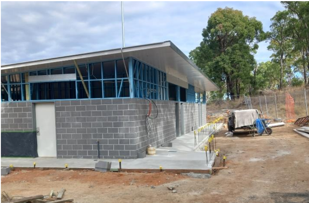
View of Northern Aspect (rear of building)
