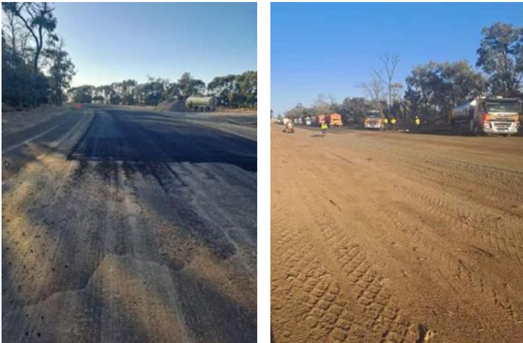
SR9 IB Bore Road
