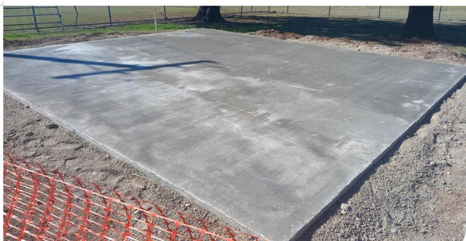
Slab for Swabbing Stall at Bingara Showground
