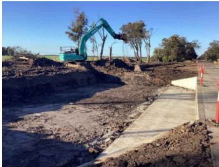
SR41 County Boundary Road, Floodway 3
