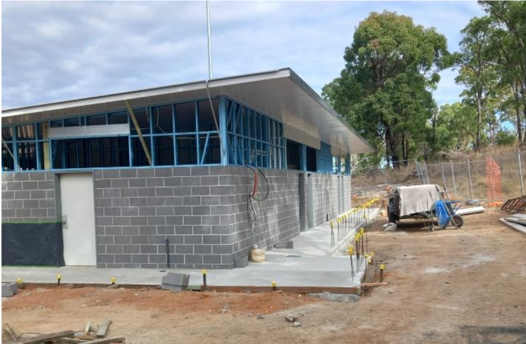
View of Northern Aspect (rear of building)
