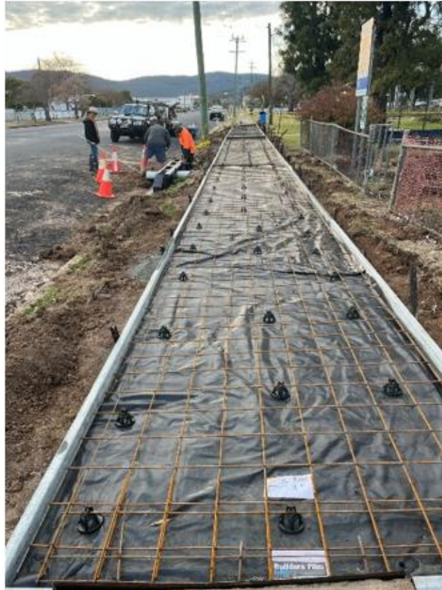
Cunningham Street footpath replacement
