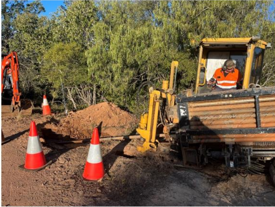
Horizontal drilling street mains
