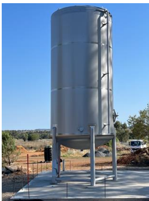
New emulsion tank at Bingara Sewerage Treatment Plant
