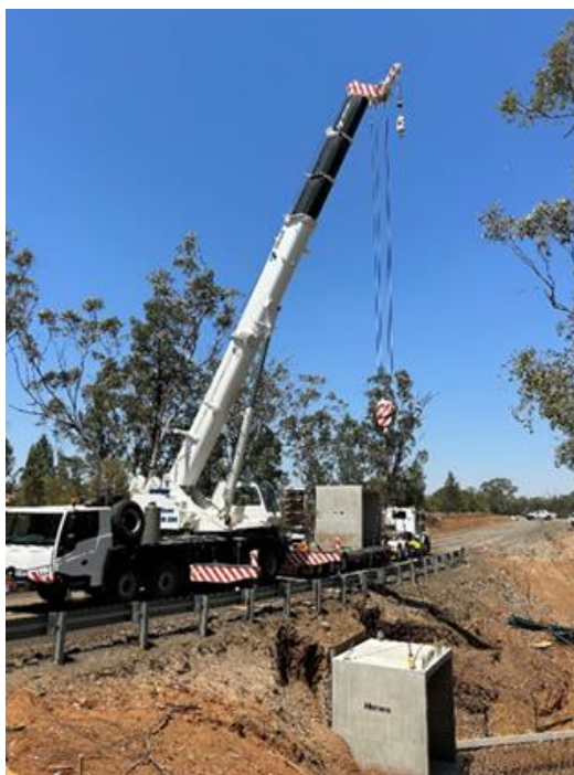
Larger box culvert units being installed at the Hollymount Rehabilitation Project.
