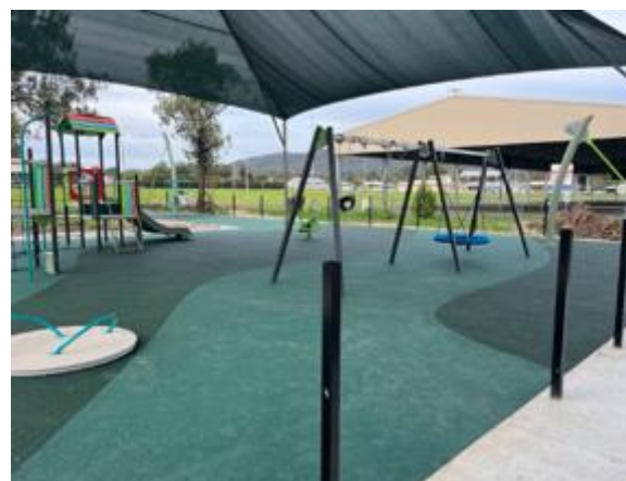
Sofffall being laid in CWA Bingara
