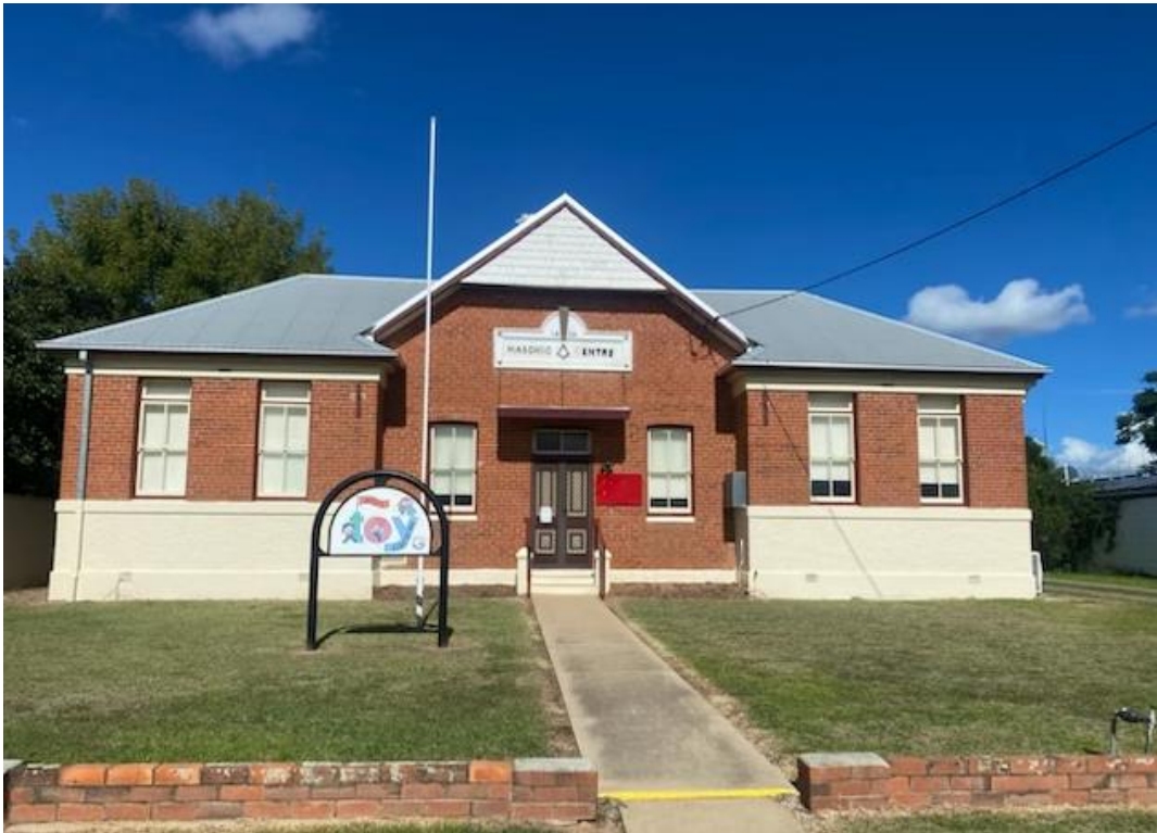
Bingara Toy Library - External painting completed
