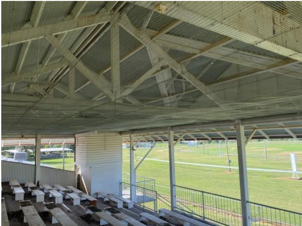
Bingara Oval – bird proofing of grandstand
