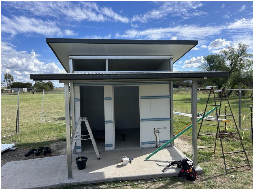
Warialda Rail Recreation Ground – new accessible amenities
