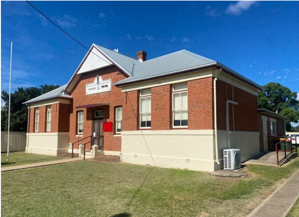
Bingara Toy Library - External painting completed
