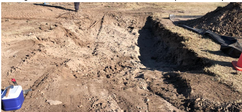
Figure 6: Fuel tank was located in northwest sector of Respite Centre facility.
