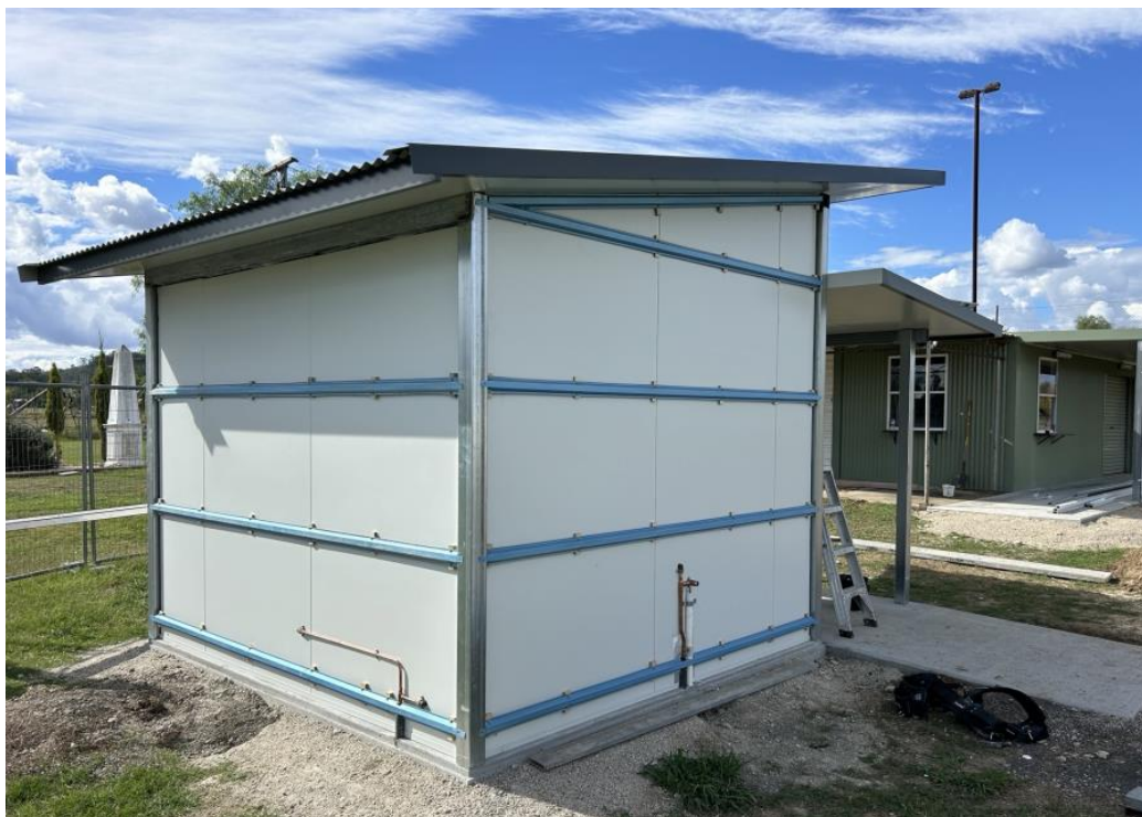
Warialda Rail Recreation Ground – accessible amenities ready for cladding
