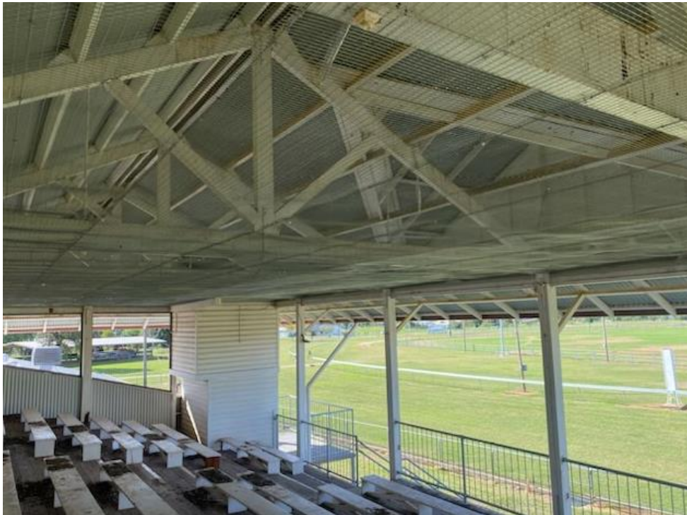
Bingara Oval – bird proofing of grandstand
