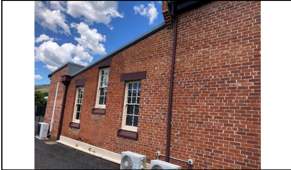
Photograph 9: Shows the eastern end of the northern elevation.
