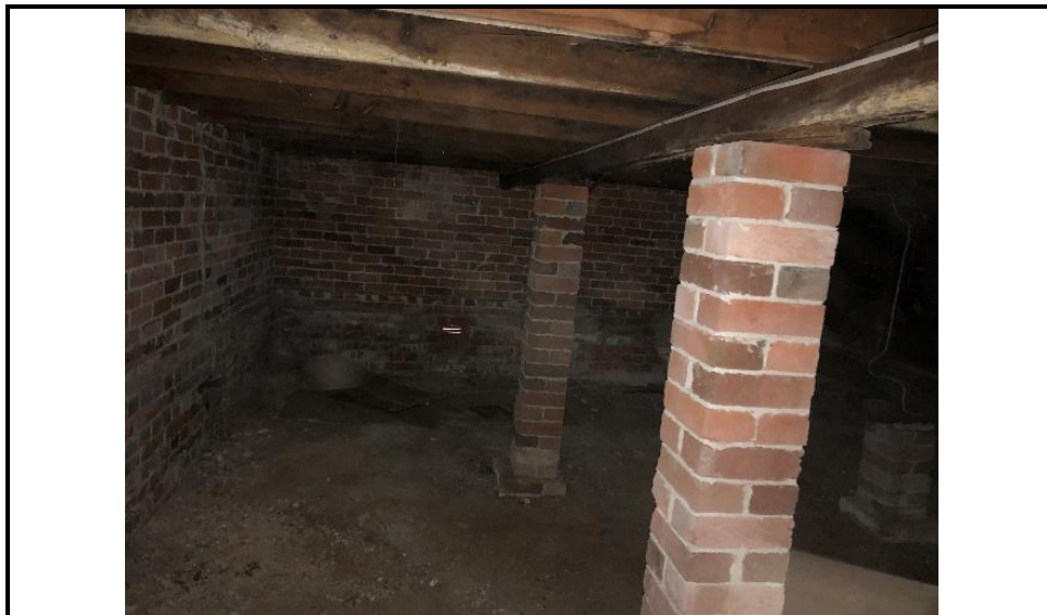
Photograph 32: Shows the sub-floor area under the stage.
