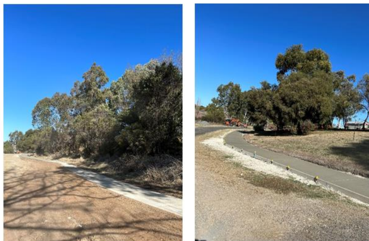
Stage 2 of the footpath completed along Reedy Creek in Warialda.
