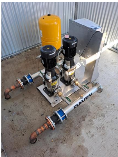
New pump installed at Gravesend Rec ground
