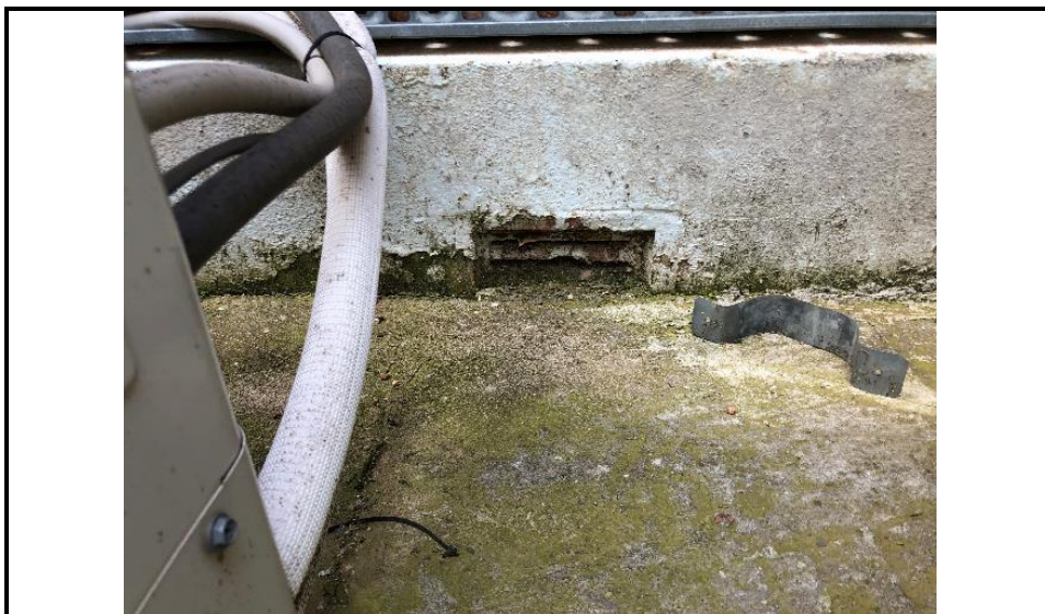
Photograph 18: Shows the wall vent under the concrete path.
