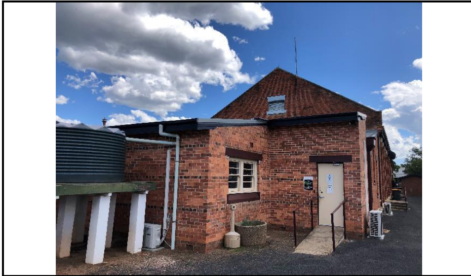
Photograph 21: Shows the rear eastern elevation.
