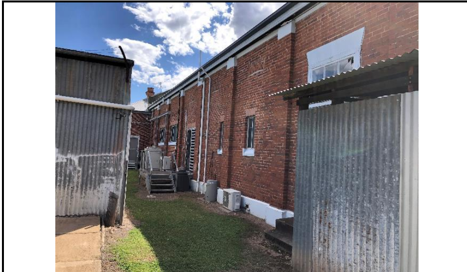
Photograph 15: Shows the southern wall elevation.
