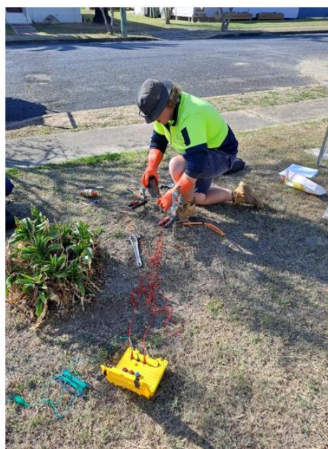
Warialda apprentice installing water meter
