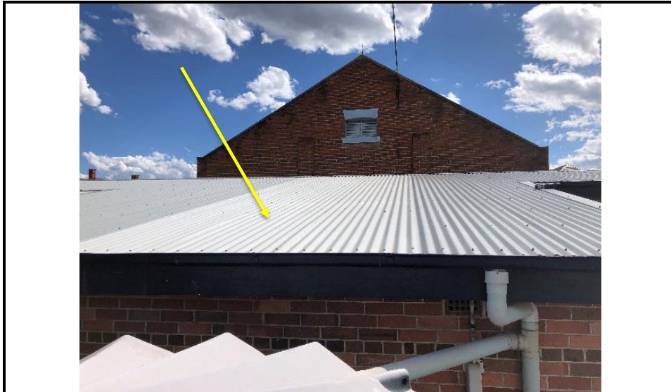
Photograph 23: Shows the new roof sheeting where the chimney was located.
