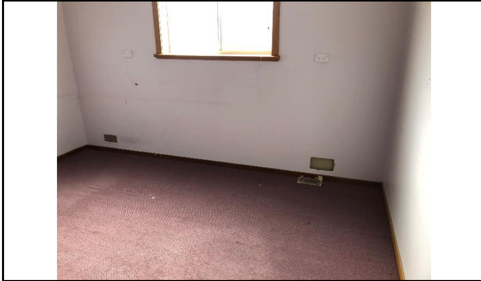
Photograph 37: Shows the wall vent in the office areas.
