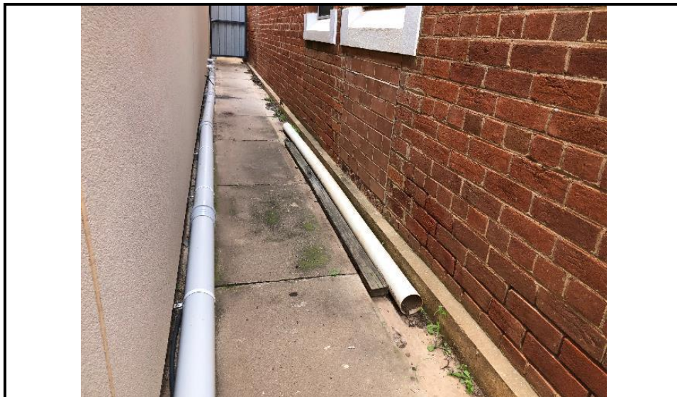
Photograph 16: Shows the western end of the southern wall elevation where all the wall vents have been covered.
