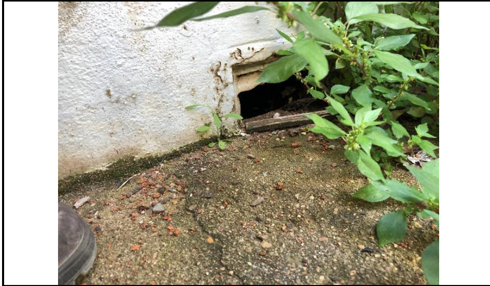
Photograph 19: Shows the wall vent under the concrete path.
