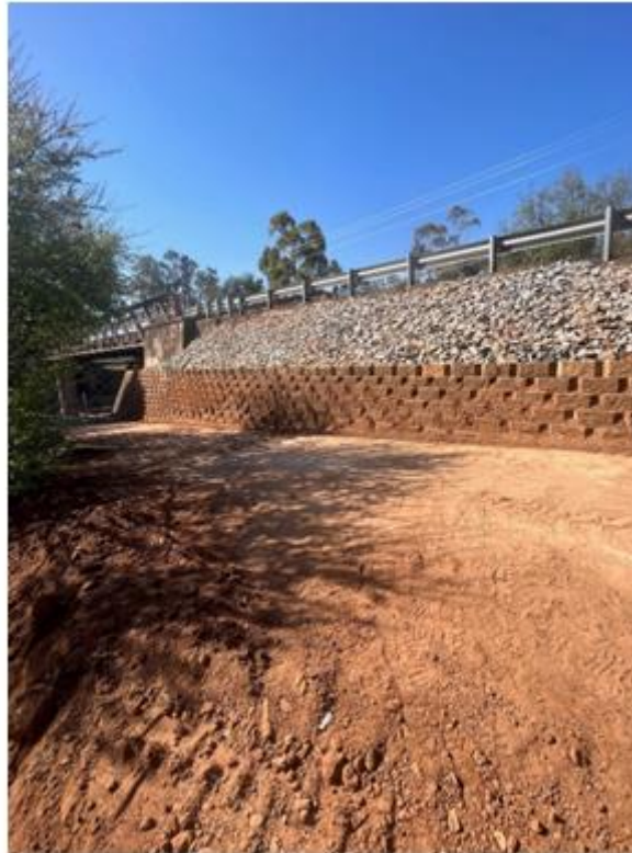
Construction works underway on the pedestrian underpass under Campbell Bridge, Bingara.
