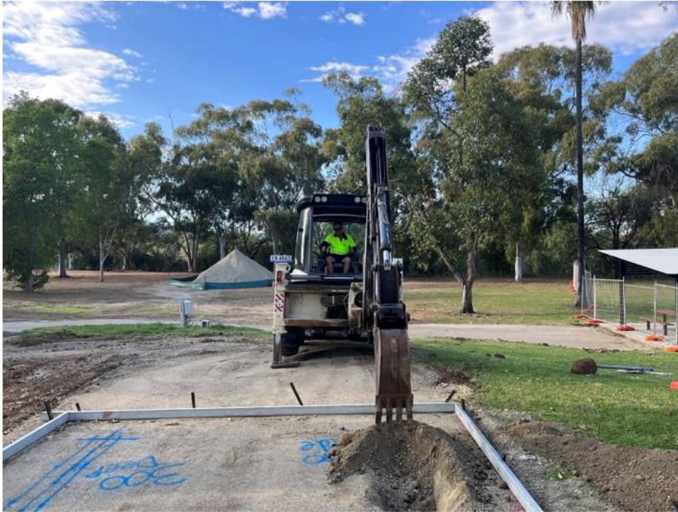
Cunningham Park earthworks for picnic shelter
