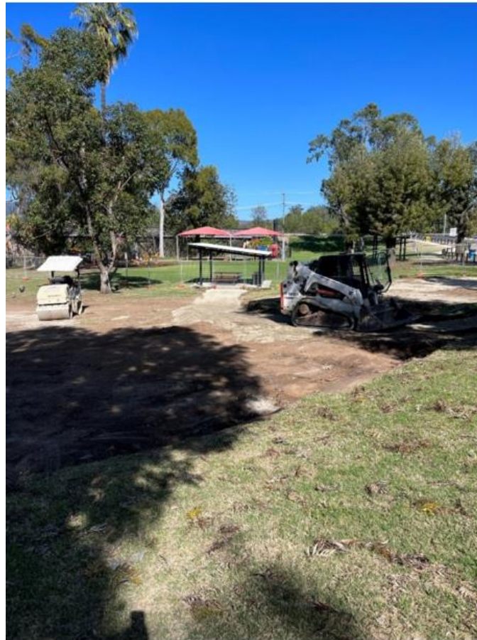
Cunningham Park earthworks
