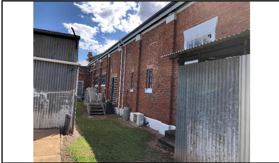
Photograph 15: Shows the southern wall elevation.
