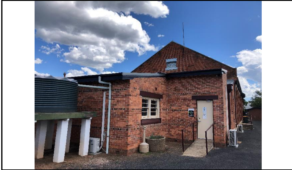
Photograph 21: Shows the rear eastern elevation.
