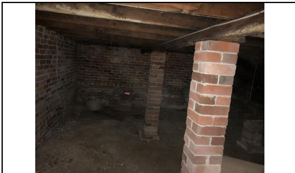
Photograph 32: Shows the sub-floor area under the stage.
