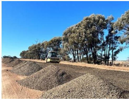
SR9 IB Bore Road
