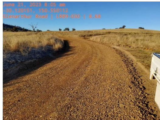
SR89 Glenarthur Road
