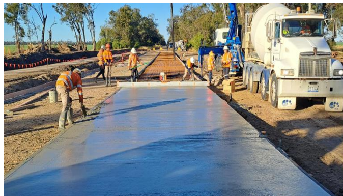
SR41 County Boundary Road, Floodway 6
